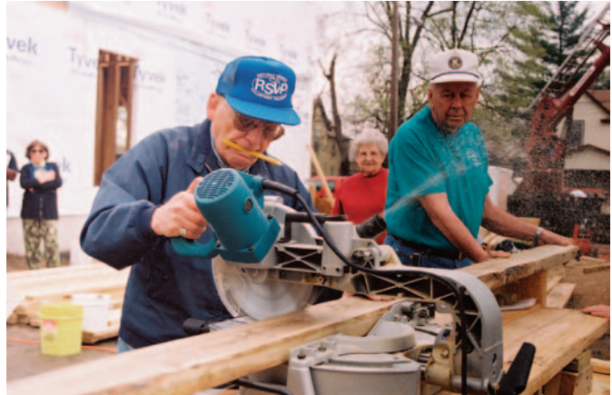
Senior Corps members building homes with Habitat for Humanity.
