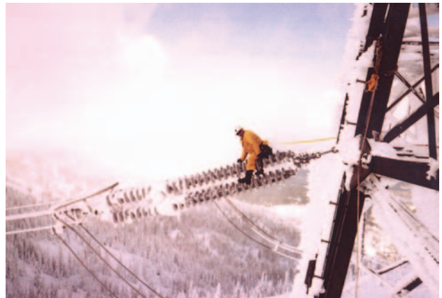
PMAs strive to provide reliable and dependable power to customers.
