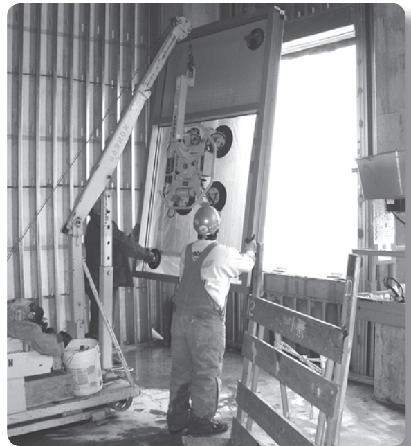
Power vacuum lifter avoids manual lifting
