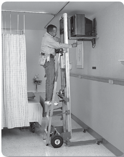
Mechanical lifts reduce the strain of holding and positioning objects
