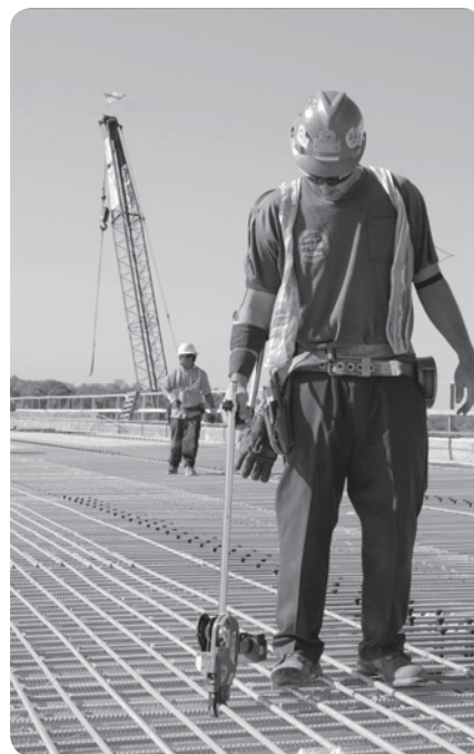
Solution: Rebar-tying tool with extension handle
