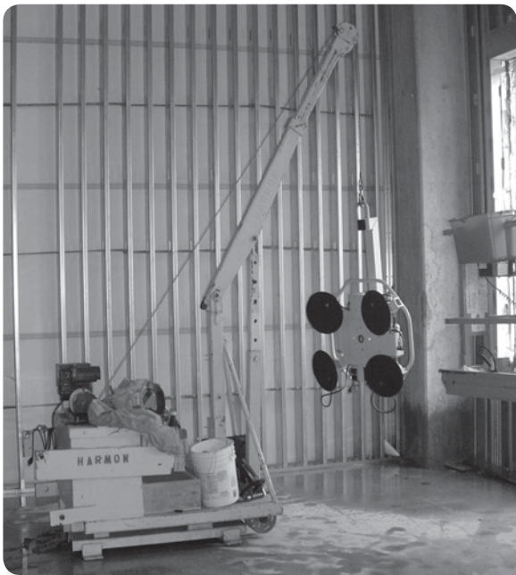
Power vacuum lifter avoids manual lifting
