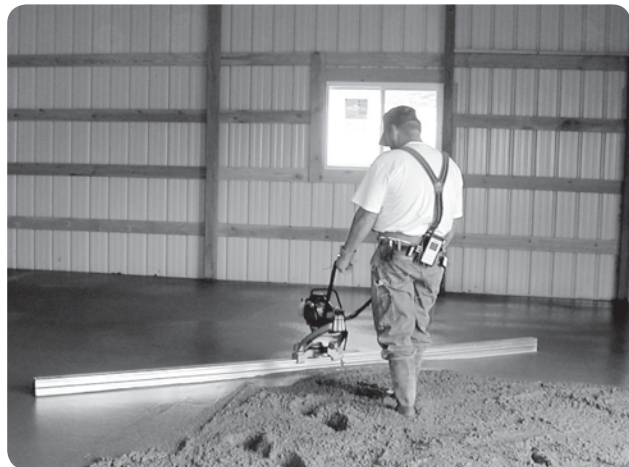
Solution: Motorized screeding
