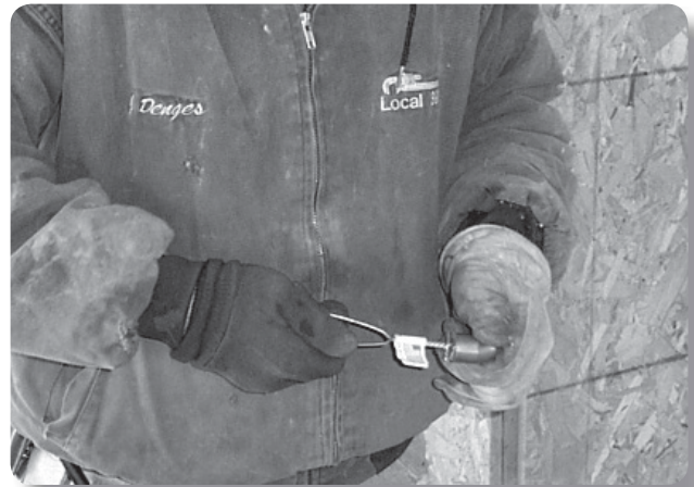
Problem: Brushing copper tube by hand
