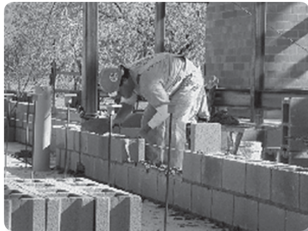
Problem: Laying standard concrete block
