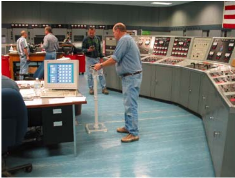
Photo 4: E-Field measurement location near VLF Transmitter control room desk
