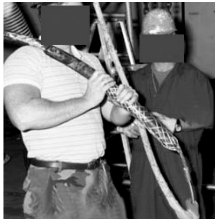
Figure 22. Cable Being Attached to Pull Rope
