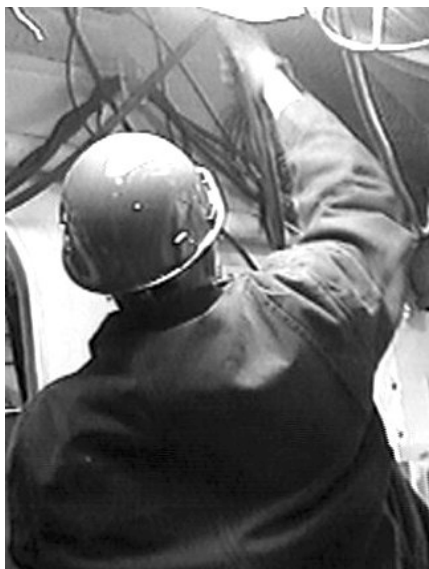
Figure 7. Cable Puller Standing, Feeding 3/4" Diameter Cable Over Head
