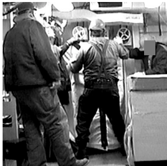
Figure 9. Sliding Equipment Off Cart
