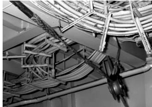
Figures 21a and 21b. Sheaves for Cable Pulling
