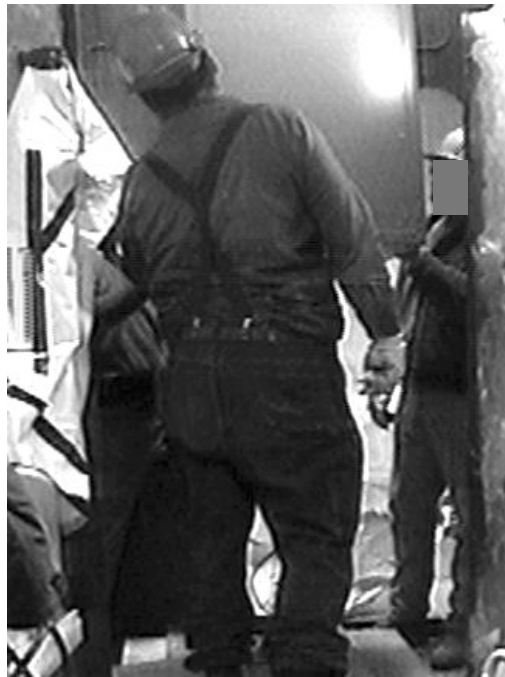
Figure 8. Lowering Equipment Through Hatch
