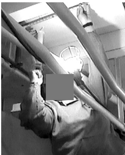
Figure 12 .Insulation Installer Measuring Insulation
