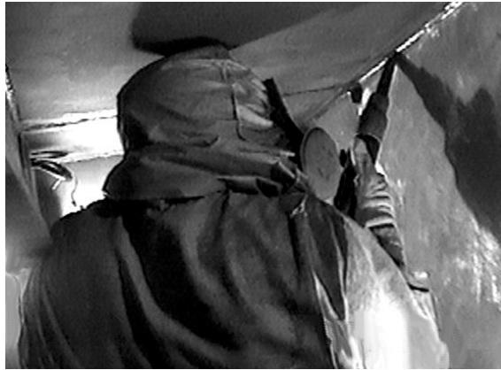
Figure 17. Tank Grinder Using Needle Gun Overhead
