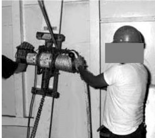
Figure 20. Cable Pulling Capstan or Winch
