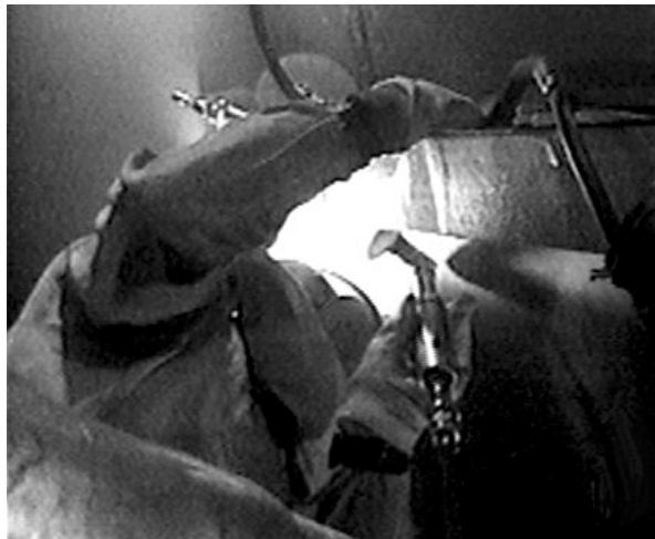
Figure 16. Tank Grinder Using 3 inch Offset Grinder
