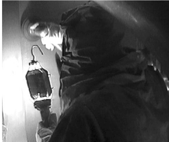
Figure 15. Tank Grinder Using 5-Inch Offset Grinder
