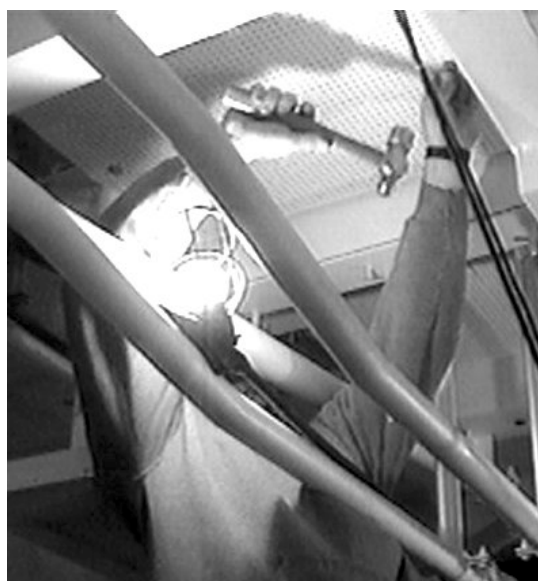
Figure 13. Insulation Installer Hammering Stud Caps Down
