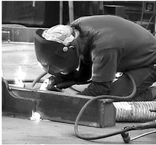
Figure 14. Panel Line Welder Wire Welding
