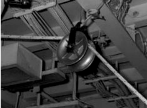
Figures 21a and 21b. Sheaves for Cable Pulling
