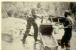
Miners "abreasting in" to a sluice.
