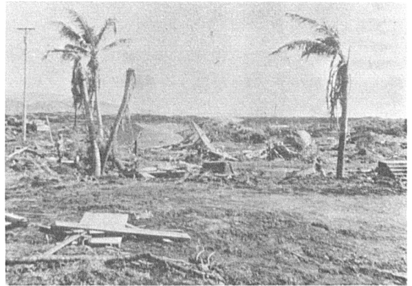
FIGURE 31.—Buildings washed off foundations and trees stripped by the tsunami of November 29, 1975, at Punaluu. Damaged palm branches indicate apparent wave height. (Photo Credit: International Tsunami Information Center)
