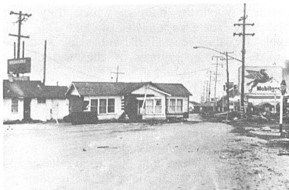
FIGURE 56.—Photograph taken in Crescent City, California, following the tsunami of March 28, 1964, showing an intersection filled with houses washed from their foundations. Photo Credit: U.S. Army Corps of Engineers.
