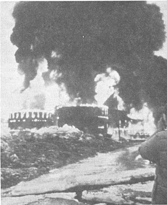
FIGURE 46.—Tank fire at the Union Oil tank farm, Valdez, Alaska, following tsunami of March 28, 1964. Photo Credit: Earthquake Engineering Research Institute.
