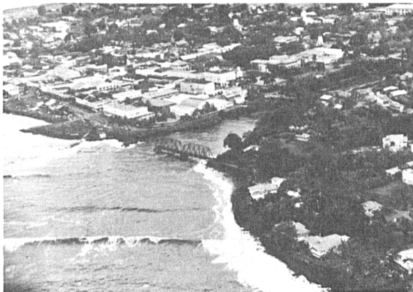
FIGURE 18.—Tsunami wave arrivals between 10 and 11 A.M. local time at Hilo, Hawaii, from the earthquake in the Aleutian Islands on April 1, 1946. Note that one span of the railroad bridge has already been destroyed by an earlier tsunami as it advanced up the Wailuku River. (Photo Credit: Univ. of California at Berkeley)
