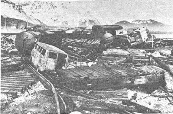
FIGURE 42.—Damage to port facilities and rail yards at Seward resulting from the March 28, 1964, tsunami. Photo credit: National Oceanic and Atmospheric Administration.
