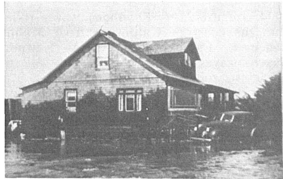
FIGURE 52.—Photo by Howard Anderson shows water height of 14.8 ft (4.5 m) at Half Moon Bay, California after the tsunami of April 1, 1946. High water reached window sills. Photo Credit: Magoon Private Collection.
