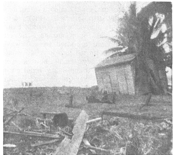
FIGURE 66.—Beach at Mayaguez, Puerto Rico, strewn with the debris of houses. Note house carried seaward by retreating wave and left stranded in the Bay. Foundation posts of houses have been destroyed by the tsunami of October 11, 1918. Photo Credit: Bulletin of the Seismological Society of America.
