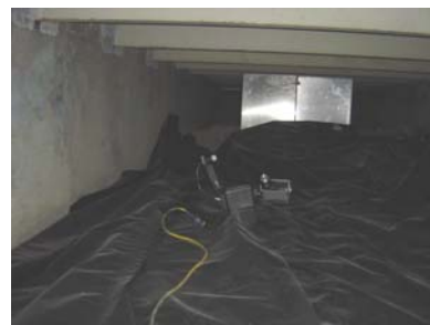
Photo 10: Crawl space in the Hale Bathhouse
