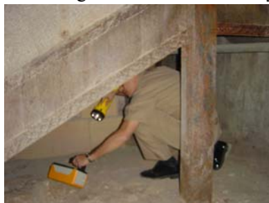
Photo 3: NIOSH investigator making radiation measurements in the Hale Bathhouse basement. This area's elevated natural background radiation level from radium-226 was identified via gamma spectrometry.
