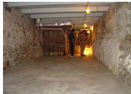
Photo 6: Radiation measurement in the Hale Bathhouse basement. A natural spring is on the left behind a wooden wall. The radiation intensity exceeded 2,500 \mu\text{R/hr} at wall contact.
