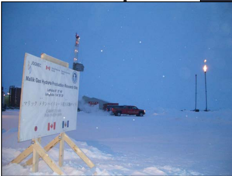
Figure 5: Methane hydrate gas still being flared six days later (March 16, 2008).
