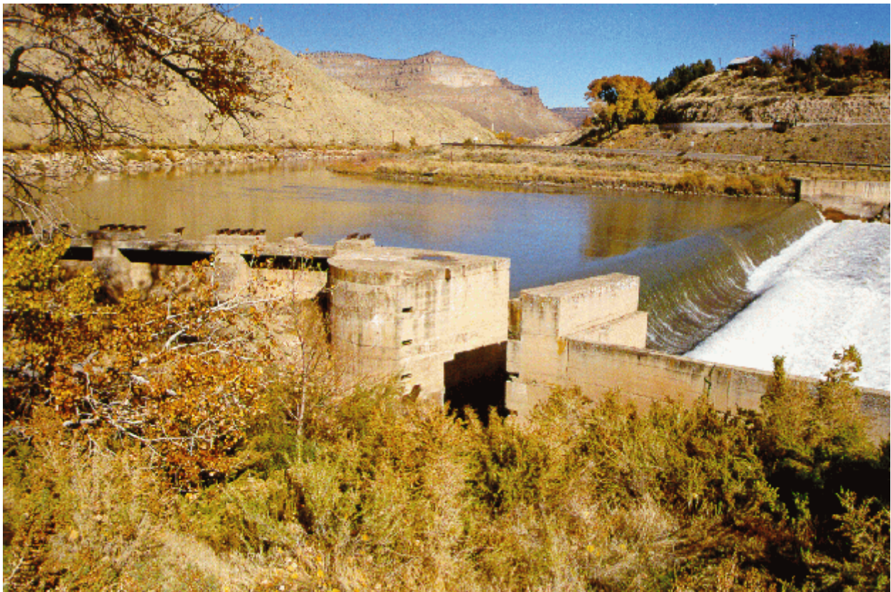
Figure 1 - Price-Stubb Diversion Dam on the Colorado River near Palisade, Colorado
