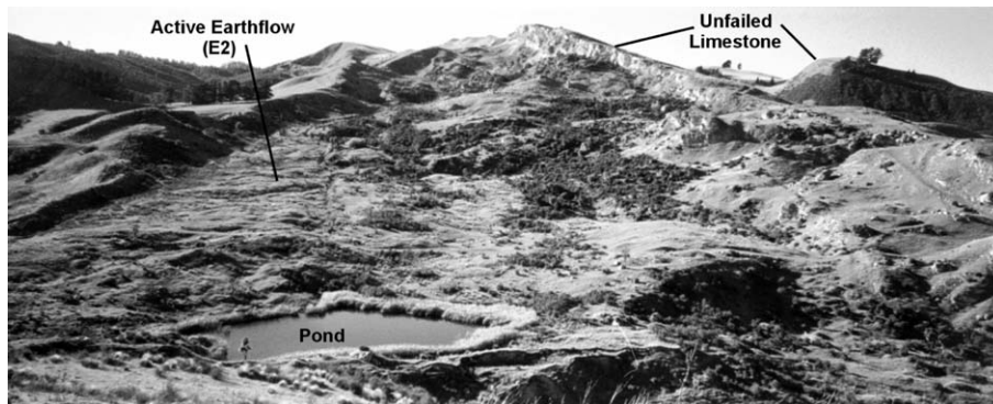
Fig. 2. Ground oblique photo of the Coringa Landslide looking north across the Motunau River. The pond in the foreground is just north of a large compression ridge at the toe of the slide. The Amuri Limestone crops out in the cliff on the true left scarp. Modern slide activity is concentrated in the earthflow E2 that lies along the true right margin of the slide and terminates just north of the pond. The surface of E2 is covered with small compression folds generally oriented east-to-west across the earthflow.
