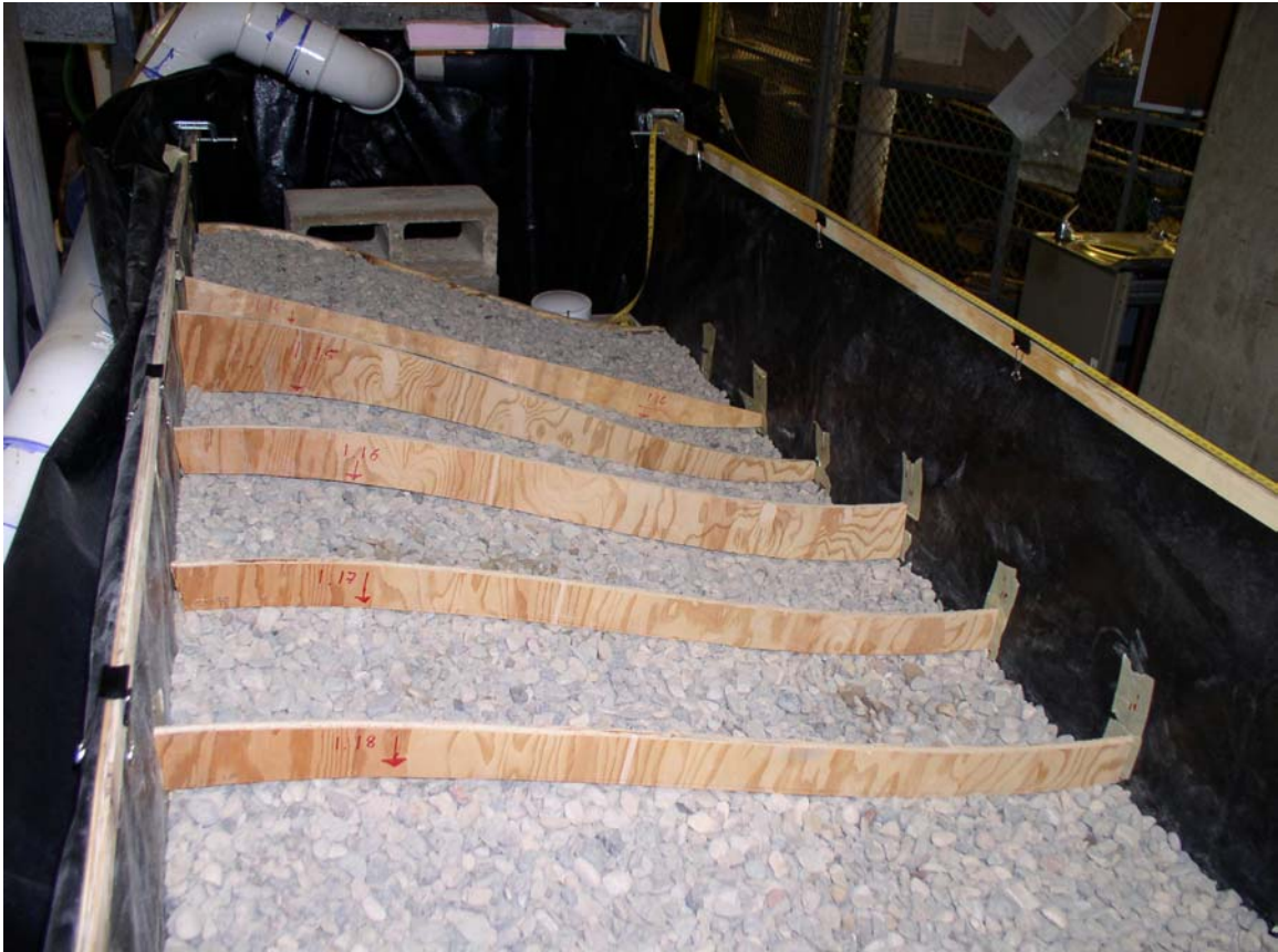
Figure 2.3: Process of pool-riffle construction using wooden molders.
