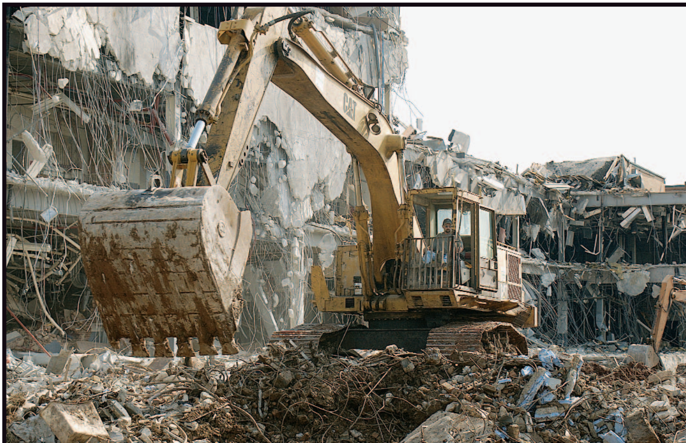
A quick and dirty solution. In traditional demolition, structures are knocked down with little regard for reusing the components. But unless a building is put together with an eye toward eventual deconstruction, demolition may be the only way to take it apart.
