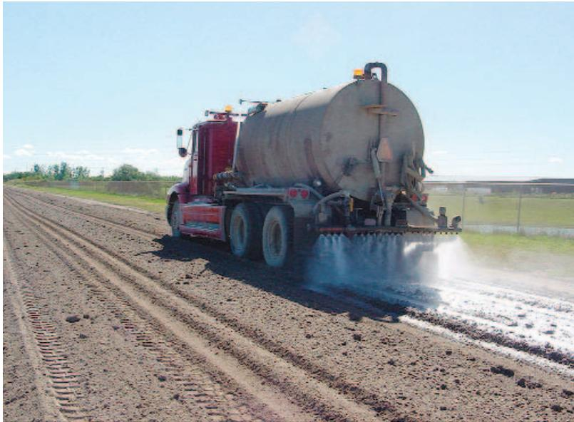
**Stopping dust safely.** A sprayer is used to apply the starch-based Dust Stop suppressant to a rural roadway.
