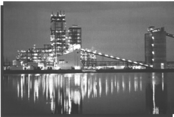
TAMPA ELECTRIC PROJECT
