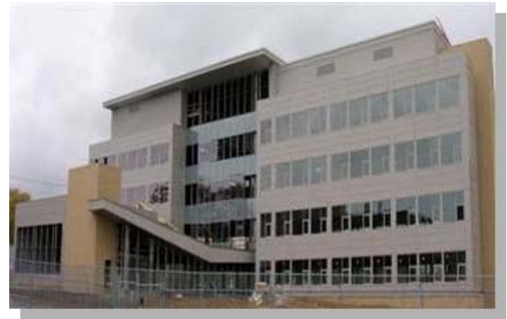
New Technology Support Facility Building Morgantown
