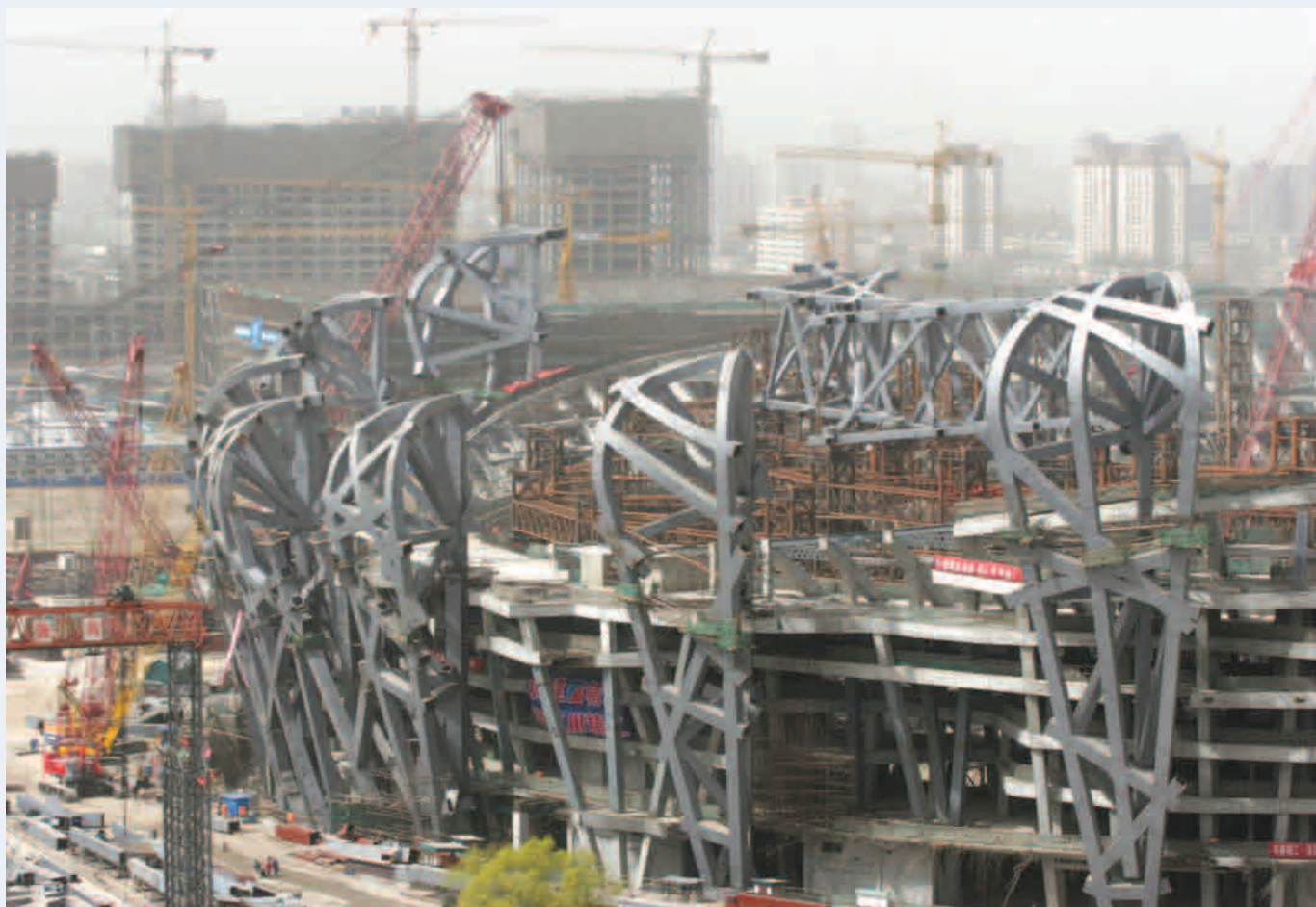
Competitive environment. Cranes add segments to the National Olympic Stadium, dubbed the “Bird Cage,” being built in Beijing for the 2008 Olympics. China’s bid to host the games included a strategic environmental assessment describing commitments such as sustainable construction.
