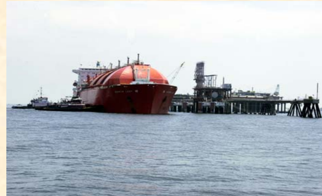
Cove Point LNG; Cove Point, MD
