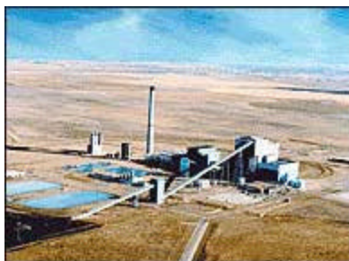
Sunflower Electric's Holcomb Station will be outfitted with a combination of innovative hardware and software to further reduce air emissions.
