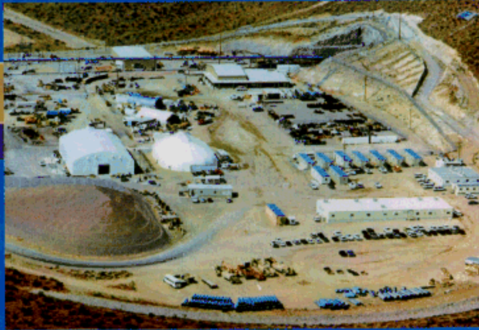
Yucca Mountain: the North Portal Area
