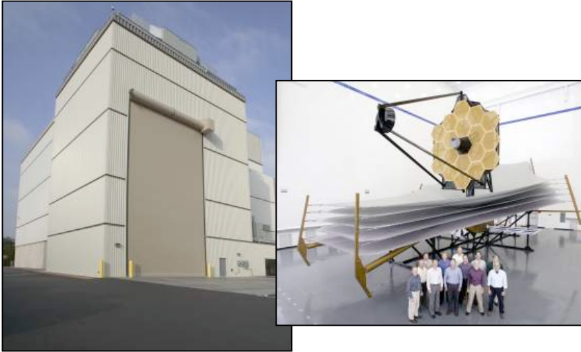
Completed new 10,500 sq. ft. Class 10K high bay for Observatory integration and test
