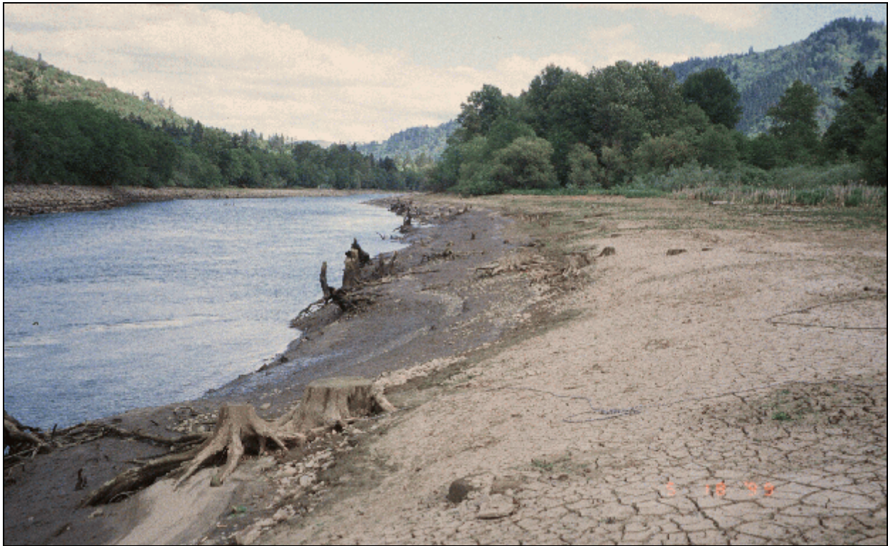
Photograph 10.—Savage Rapids Dam, Rogue River Basin Project, Oregon. View upstream showing the surface of the south bar as exposed while the reservoir pool was low during stoplog installation. The south bar consists of fine sand and silt, based on earlier explorations by McLaren/Hart (1998) and is underlain by bedrock of the Applegate Group at depths ranging from 6.5 to 14.8 feet in five test borings drilled at this site. (Reclamation photograph by Richard Link; May 18, 1999.)
