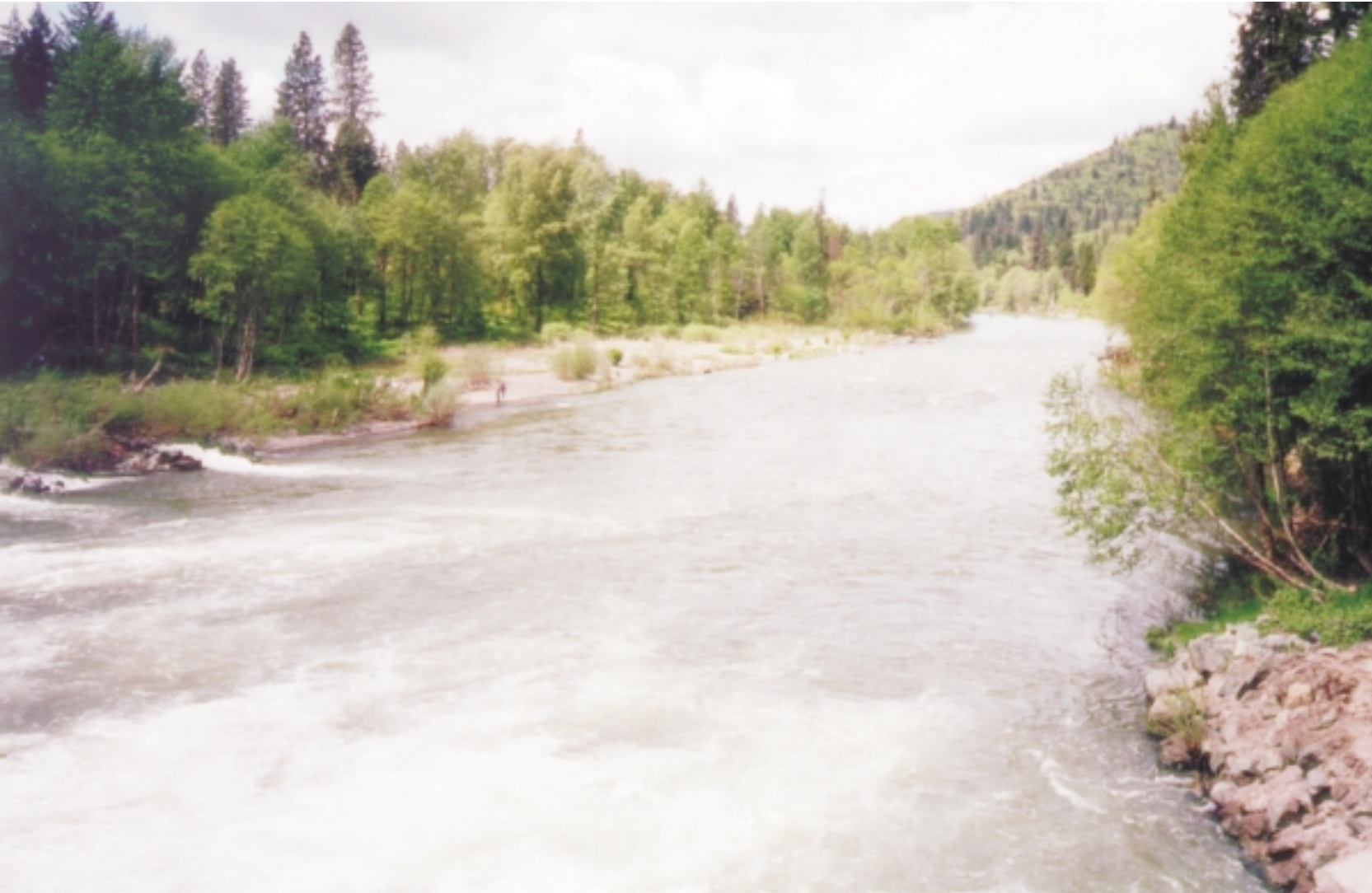
Figure 25. - Looking downstream from Savage Rapids Dam at the proposed location of the two pumping plants which would supply water for the Grants Pass Irrigation District. One plant would be constructed on each side of the river.
