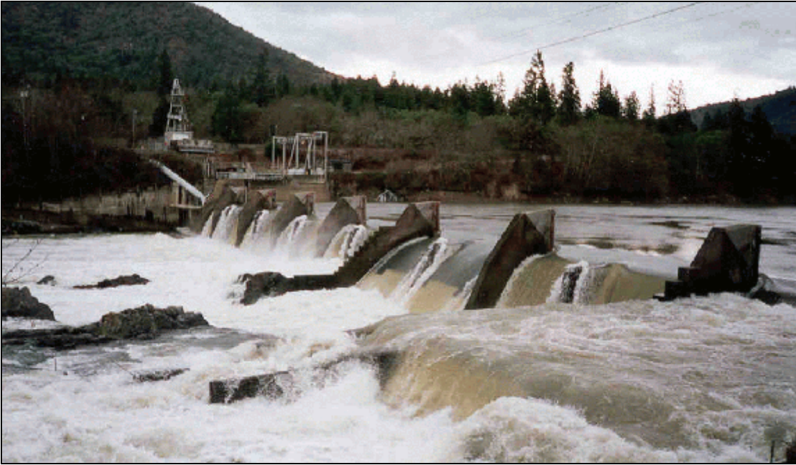
Figure 2.—View of Savage Rapids Dam, located on the Rogue River in southwestern Oregon, 5 miles upstream from Grants Pass. Photograph by Tim Randle on February 23, 1999. The mean-daily flow on this date was 7,400 ft 3 /s (U.S. Geological Survey gauge at Grants Pass, Oregon).
