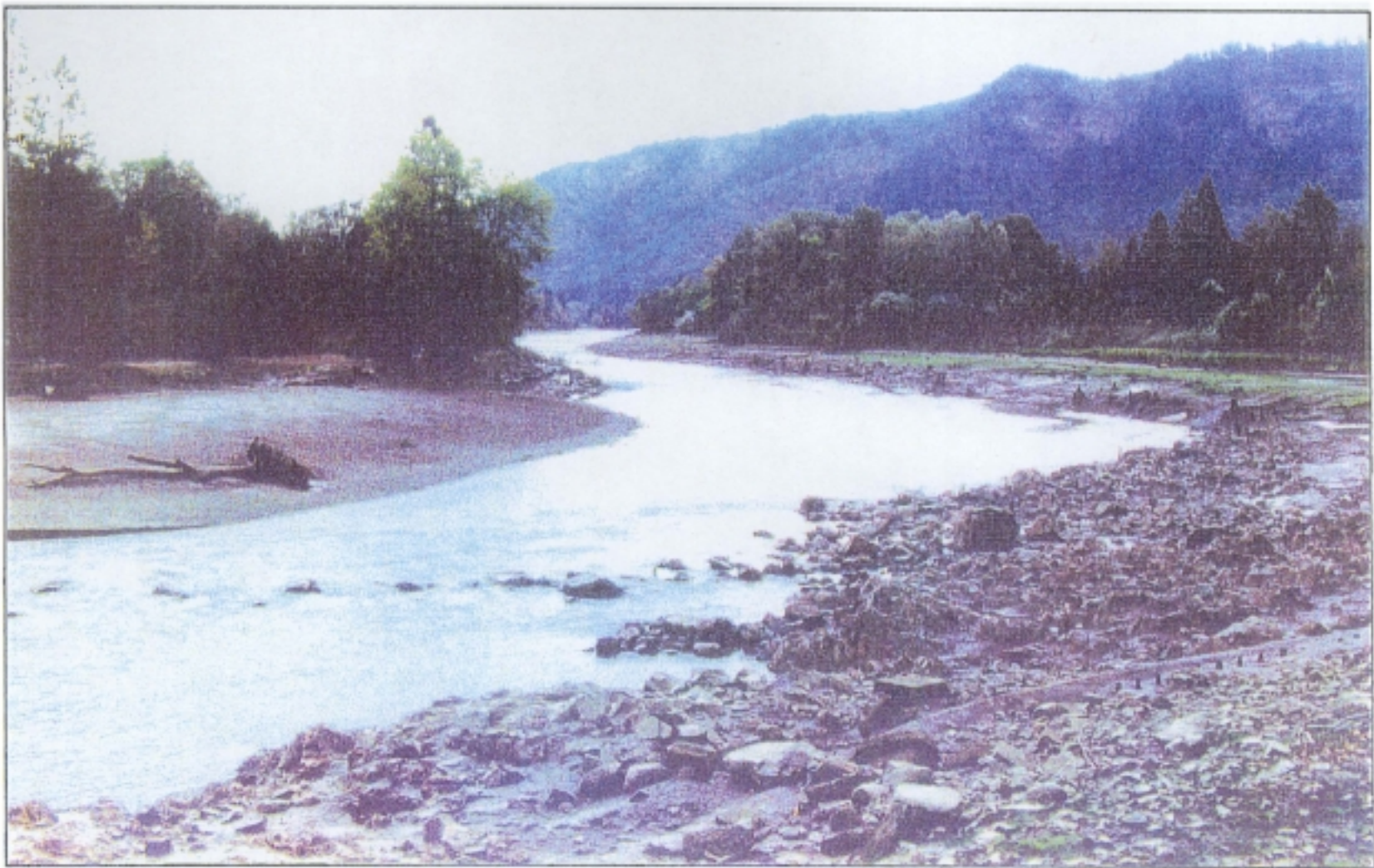
Figure 10. - After the stoplogs are removed following the irrigation season, riverine conditions exist upstream from the public boat ramp in Savage Rapids Reservoir.
