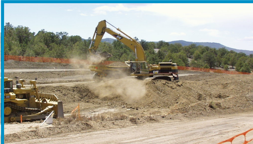
Excavation operations on the inlet conduit sleeve.
