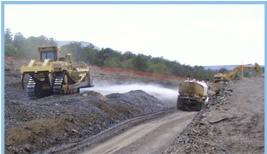
Water truck applying water for dust control.
