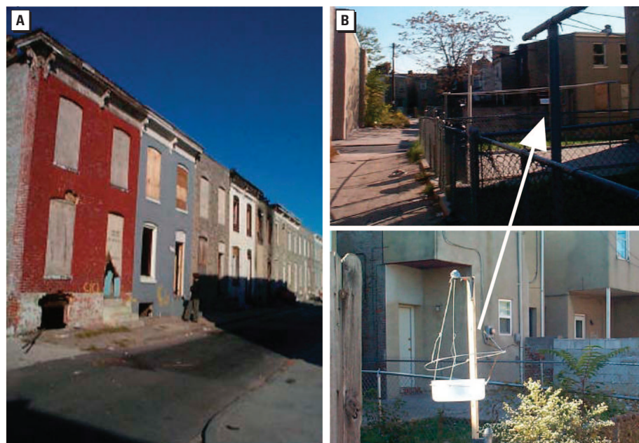
Figure 2. Before demolition, site 1. (A) Row houses. (B) Dust-fall collection apparatus with arrow pointing to another view of the same sampling location.
