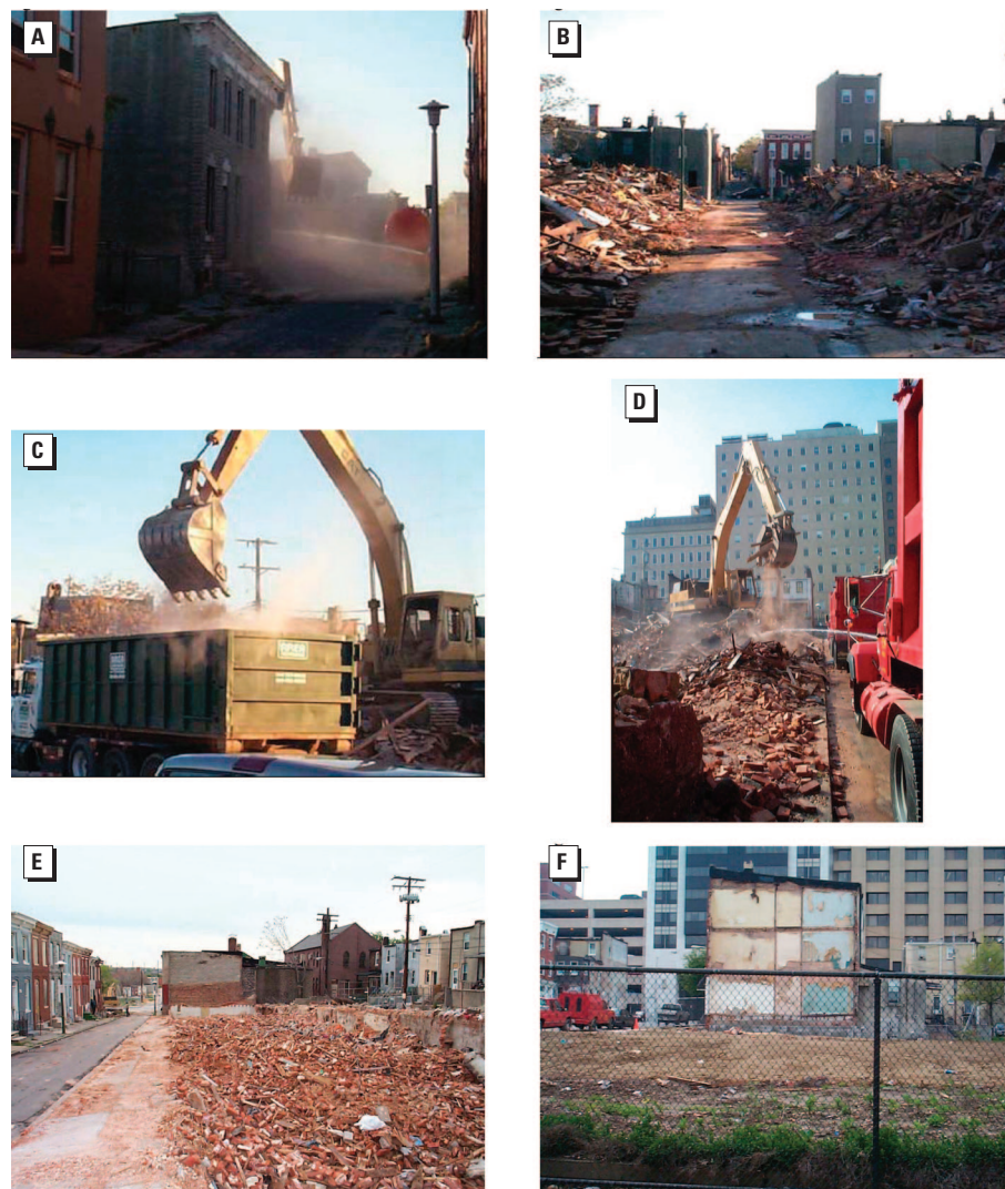
Figure 3. Demolition in progress. Site 1: (A) during demolition; (B) after demolition and before debris removal; and (C) debris removal. Site 2: (D) debris removal; (E) after debris removal; and (F) vacant lot.
