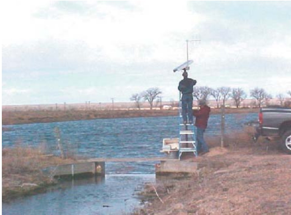
Installation of a radio-controller unit on the Sandhill measurement site of the South Platte Ditch Recharge System.
