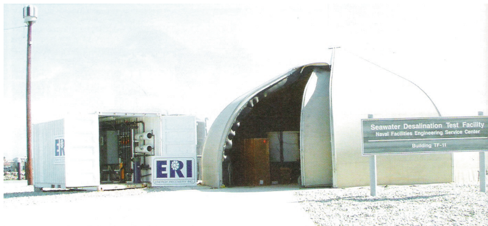
Site of the coming Affordable Desalination Collaboration's seawater reverse osmosis demonstration.
