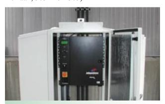
Proton exchange membrane (PEM) fuel cell system. An outdoor enclosure houses the Avista Labs, Inc. Independence 1000 fuel cell, associated controls, and six hydrogen fuel cylinders. The fuel cell is rated at 1,000 watts at 54 volts. This system provides about 30,000 watt-hours of backup power for the Pole Hill Powerplant communication system.
