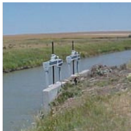
The Townsite Lateral headgate in North Canal.
