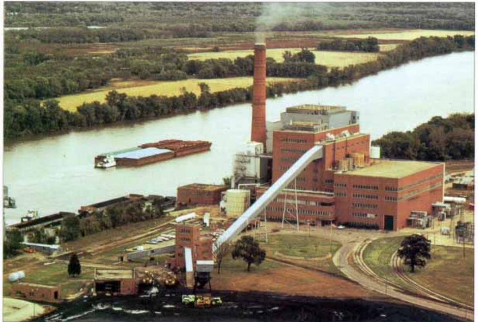
Illinois Power's Hennepin Unit No. 1 is the demonstration site for the GR-SI process on a tangentially-fired pulverized coal unit.
