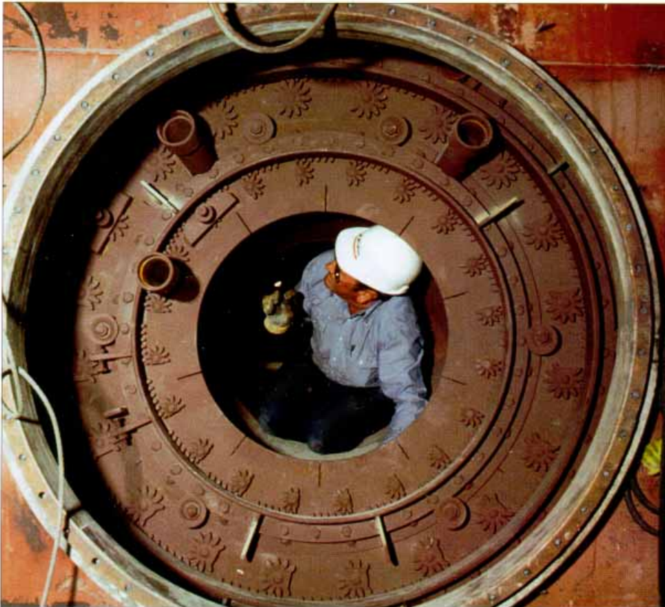
The mounting shroud for the low-NO x burner is being checked during installation in the boiler wall at Cherokee Unit No. 3.
