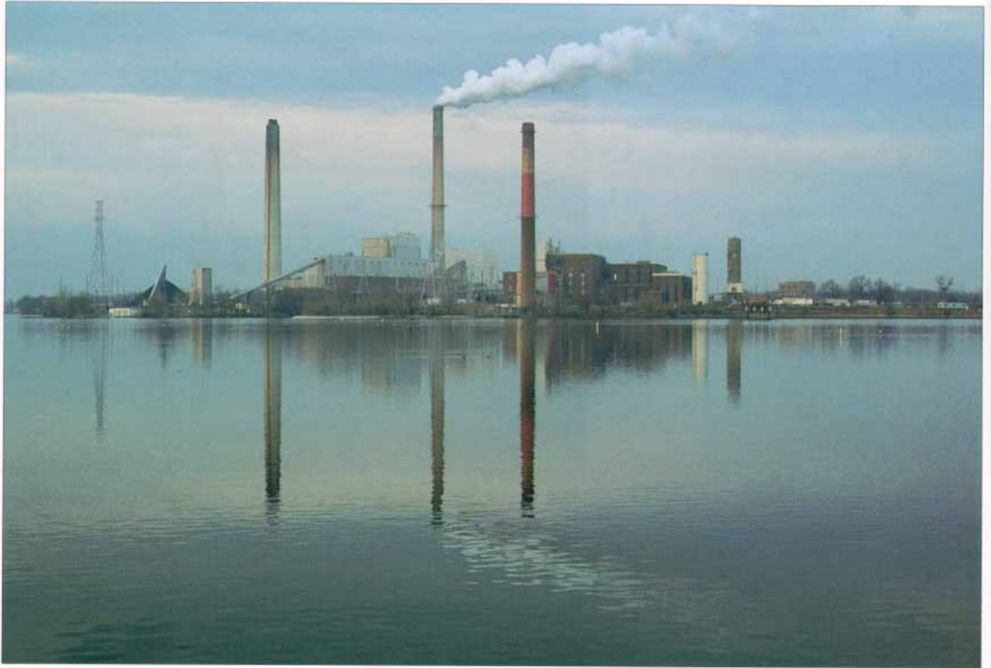
City Water, Light and Power Company's Lakeside Unit 7 is the demonstration site for GR-SI technology on a cyclone-fired boiler.
