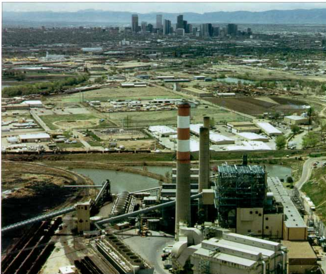
Public Service of Colorado's Cherokee Station Unit No. 3 is the test site for the GR/Low-NO x Burner technology demonstration. It burns low-sulfur western coal. The city of Denver, Colorado is in the background.
