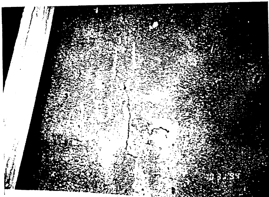
Photo #11 - View of crack in concrete column on north quadrant at elevation 80' behind the ladder. The crack is hairline and ends at elevation 102'.
