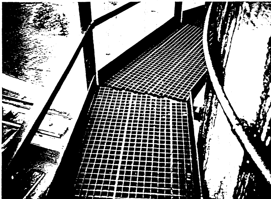
Photo #20 - View of platform at top of chimney. The platform is in safe and sound condition.
