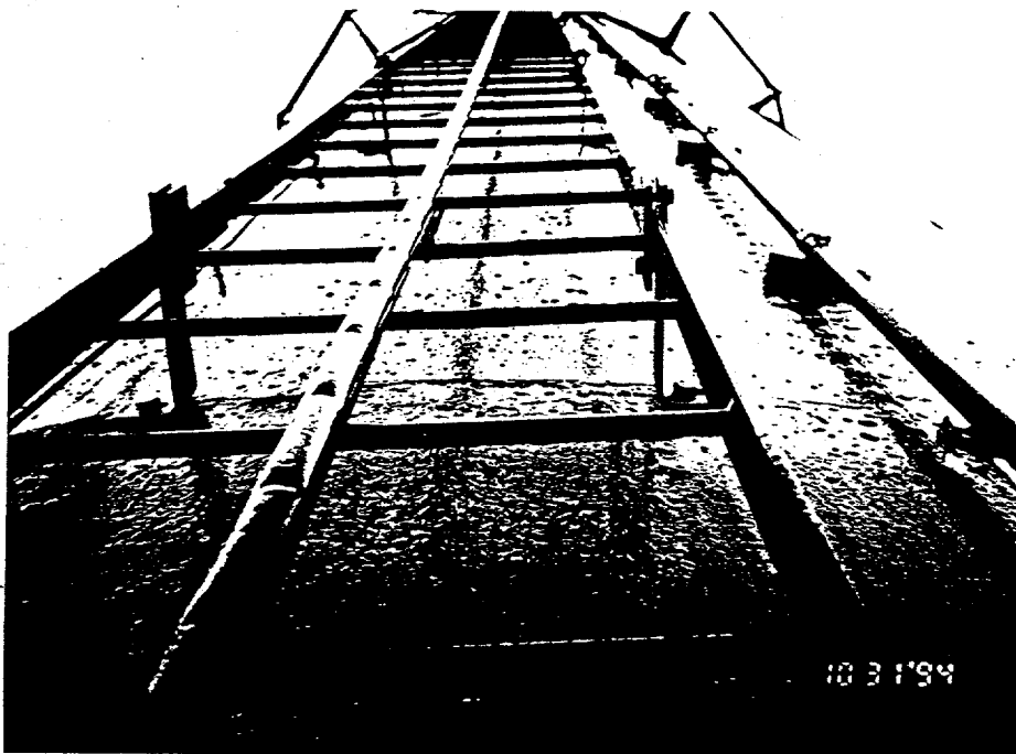
Photo #18 - View looking up ladder system from elevation 220'. The ladder is solid and sound. Minor rusting and staining were noted.
