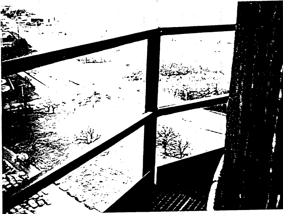
Photo #25 - The handrails and support steel of the top platform is stained and rusting freely.
