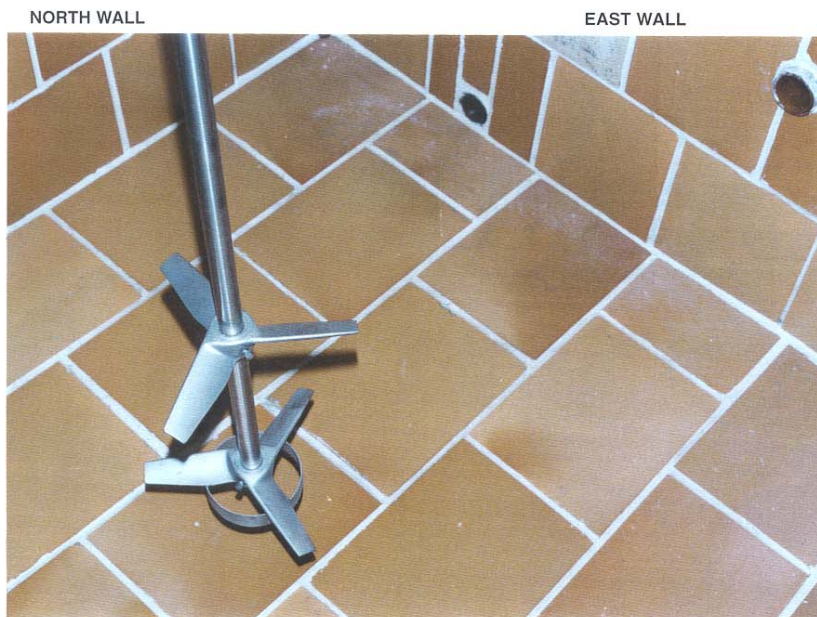
Photo 3.11 Concrete foundation slab with first row of tile installed.
