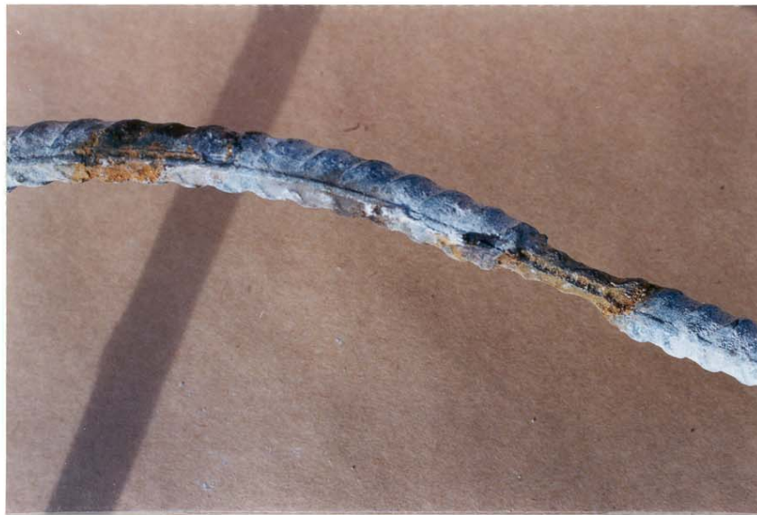
Photo 3.4 Dowel "A" close-up.
