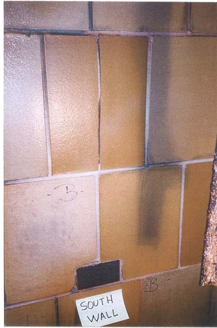
Photo 1.5 Split tile and refrax plug in spray impact area, photographed in October 1995 after 7,986 hours of operation.
