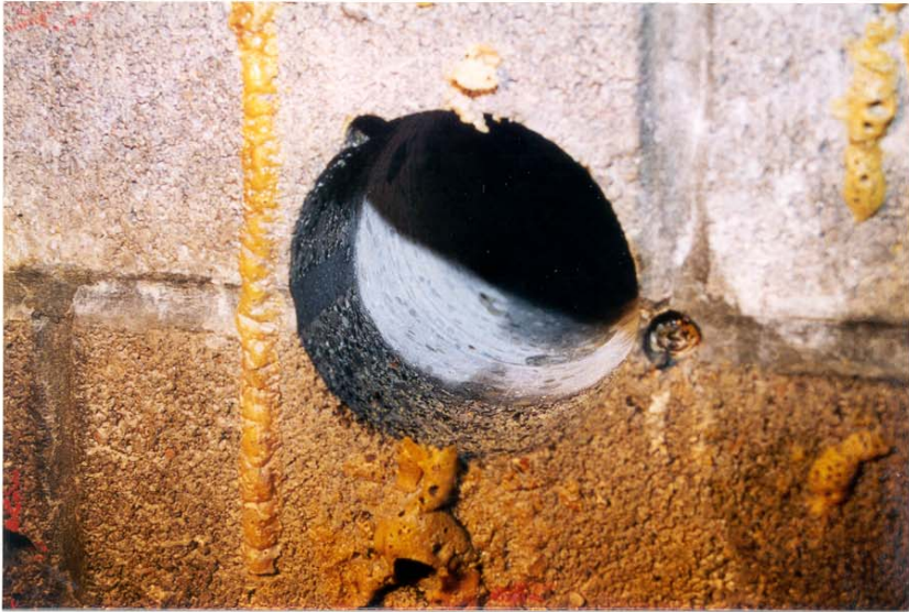
Photo 2.22 Core hole S7-4, sealant used to plug drilled holes is evident.
