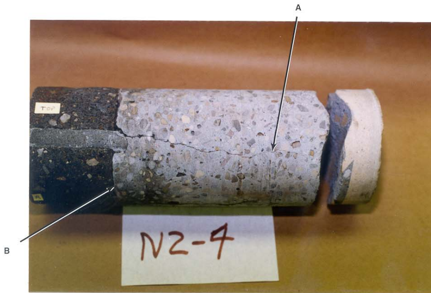
Photo 2.1 "A" shrinkage or thermal crack starting at a vertical mortar joint which protruded into the concrete. Crack "B" see photo 2.2.
