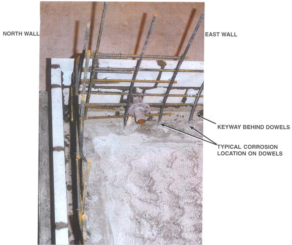
Photo 3.9 Concrete foundation slab during construction.
