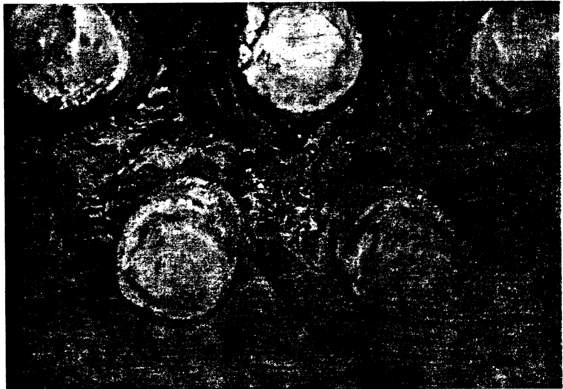
Figure 38. Close up of plugged area between rows 2 and 3 from the bottom of the hot-end tube bank. Area between the tube rows is totally plugged.
