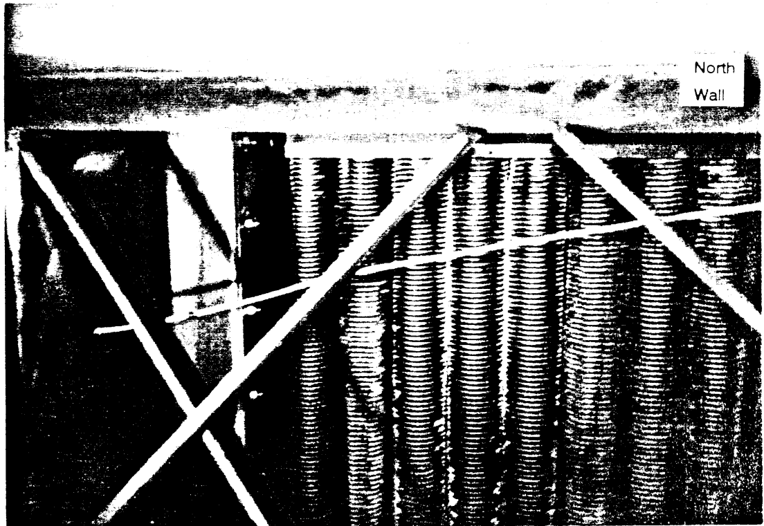
Figure 18b. End of Phase II testing -- Bottom side view of cold-end outlet heat pipes at outside (north) wall. Heat pipes show slightly more fouling than at the beginning or middle of the Phase I testing.
