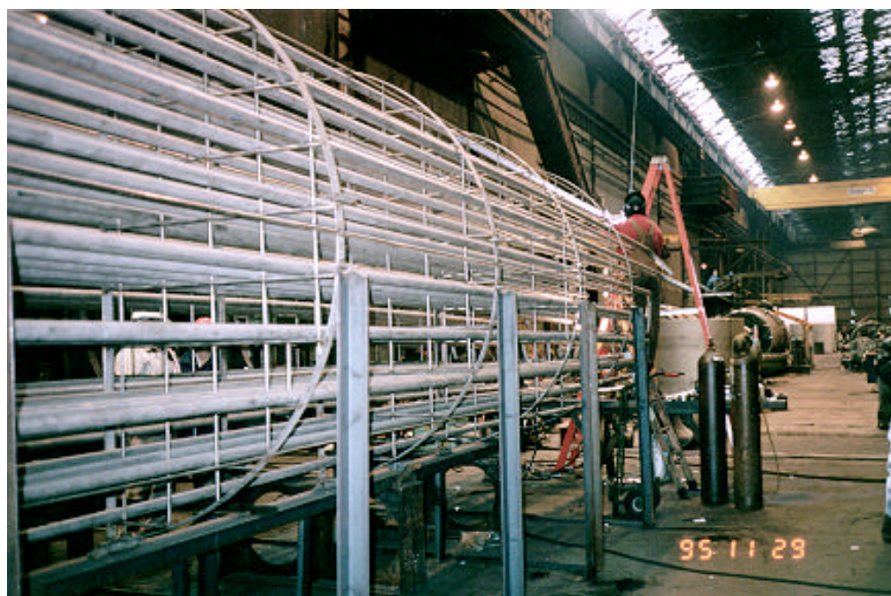
Figure 2 - Fabrication of Internal Heat Exchanger
