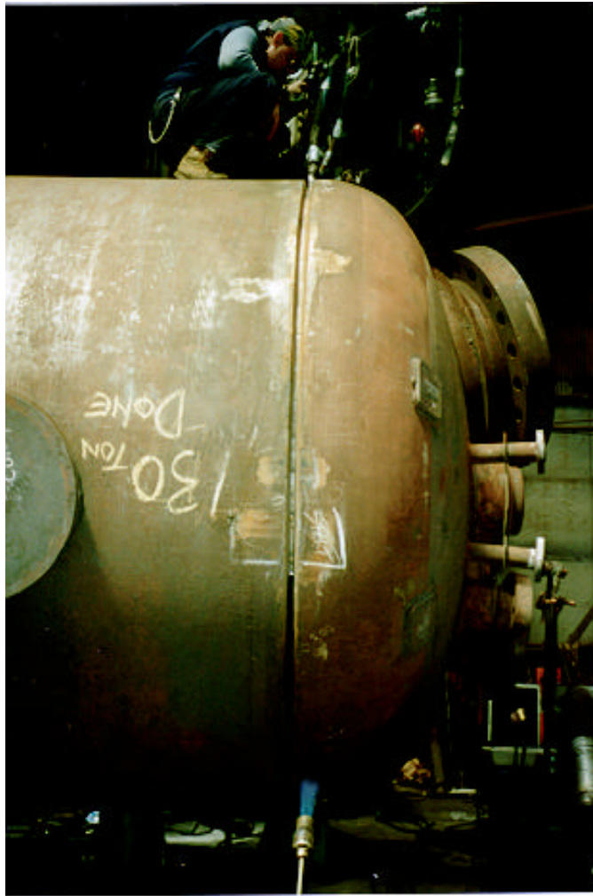
Figure 5 - Welding of Head-to-Shell Seam
