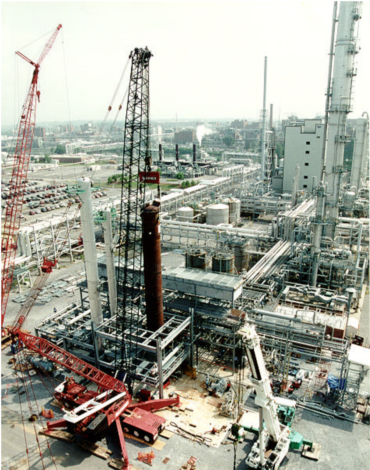
Figure 8 - Reactor Installation
