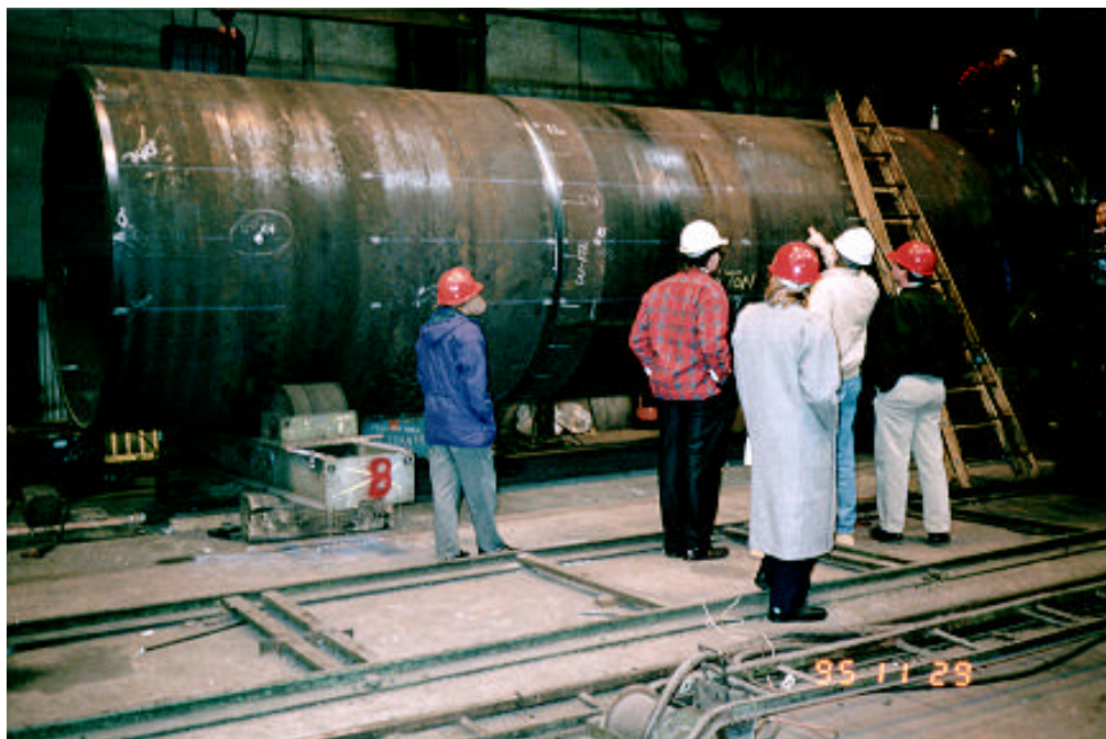
Figure 1 - Fabrication of Reactor Shell
