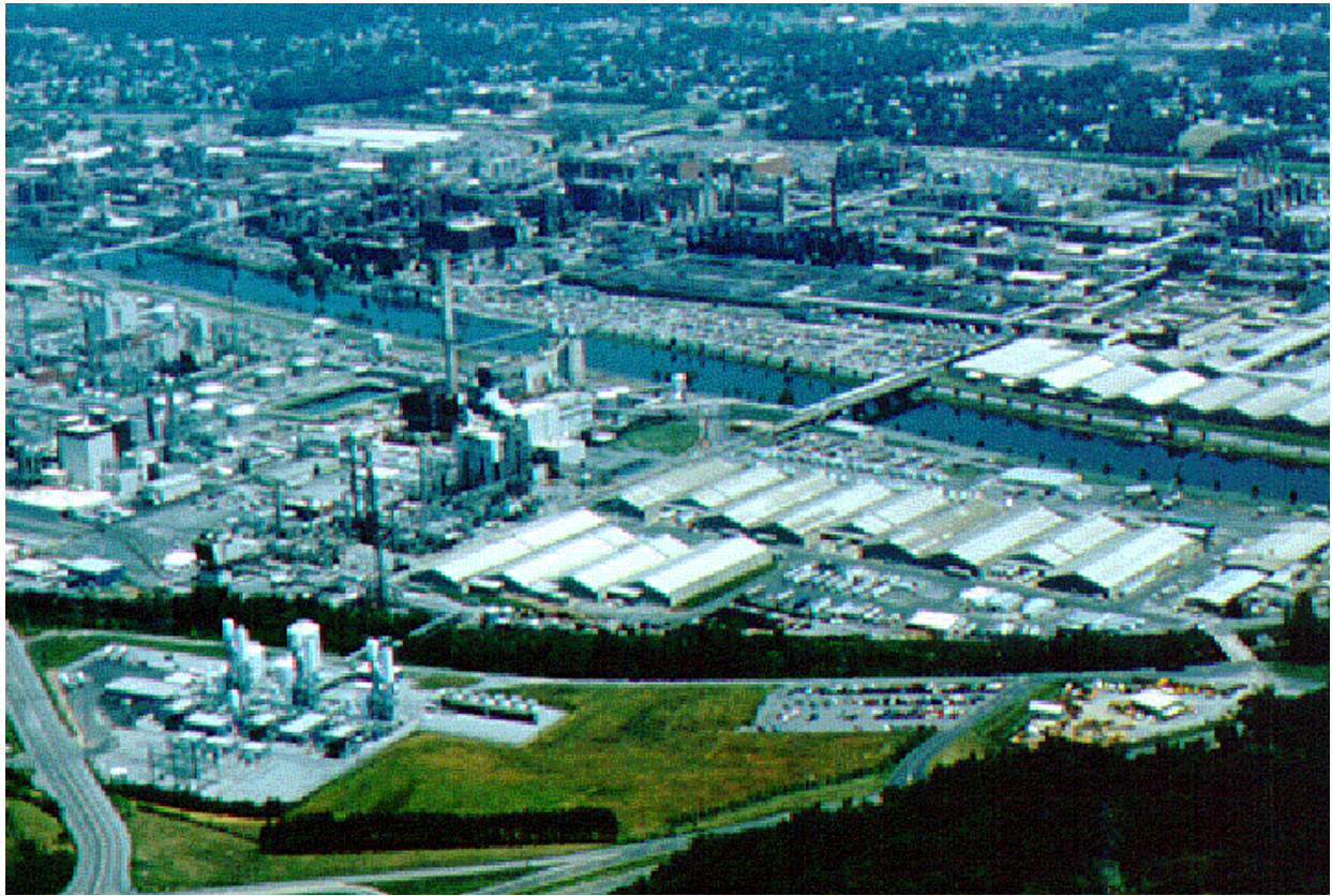
Aerial Photograph of Eastman Chemicals-from-Coal Complex
