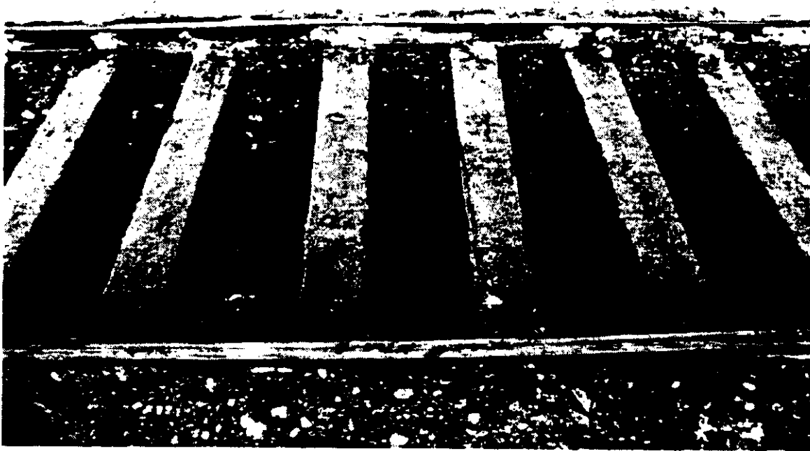
PHOTOGRAPH 5. Close-up view of the railroad bed after some of the contaminated gravel was removed.
