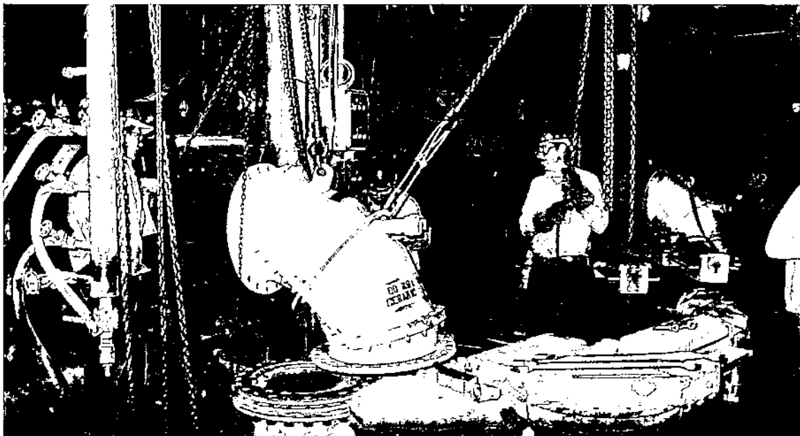
Figure 4-10 A ceramic-lined coal elbow is installed on the burner front. The ceramic lining resists the erosive effects of the pulverized coal.
