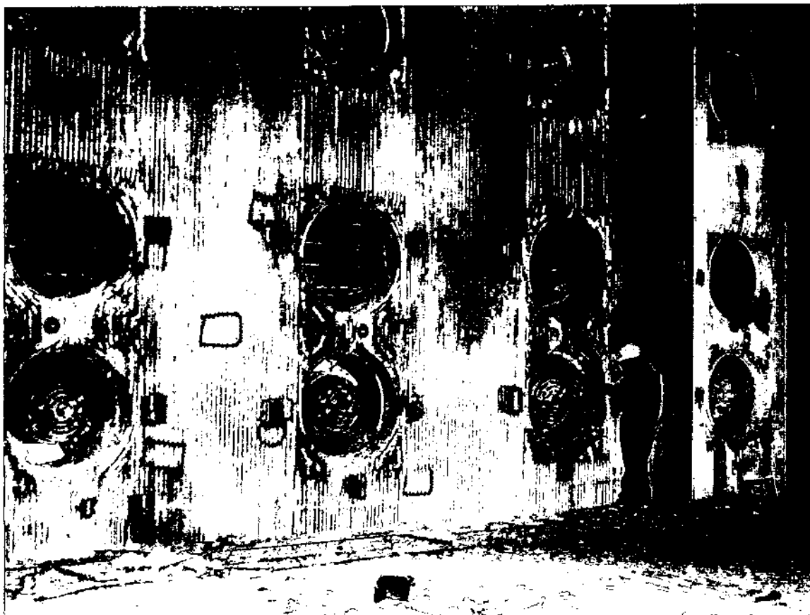
Figure 4-13 A wall of LNCB™ burners viewed from inside the furnace prior to inversion of every other lower level burner and NO x port. Each burner and NO x port function as a unit and constitute one Low-NO x Cell™ burner.
