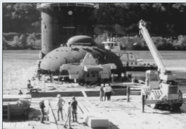
Worker's ready to unload the prefabricated pressure vessel
