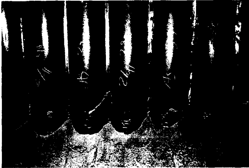
Figure 16-15. Erosion Patterns Initiating from the Membrane in Combustor A (February 1991 Outage).
