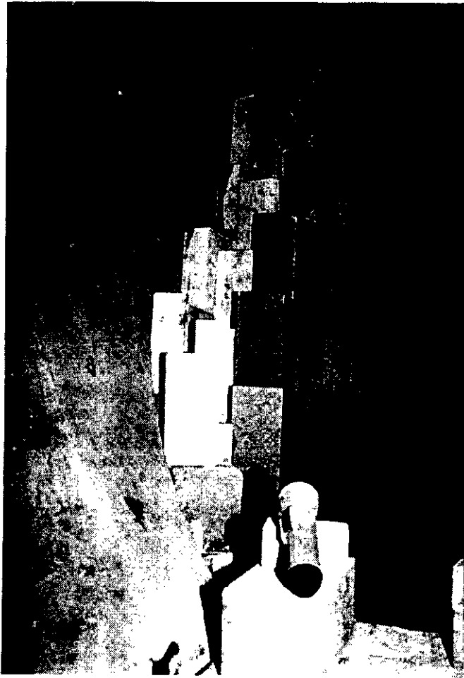
Figure 16-33. Brick Reconstruction in Loop Seals (January 1989 Outage).
