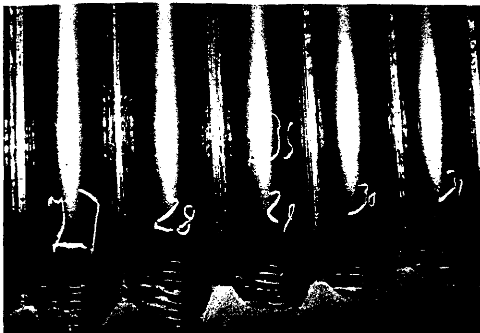
Figure 16-11. Worn Weld Overlay at Refractory/ Water-wall Interface in Combustor B (February 1991 Outage).
