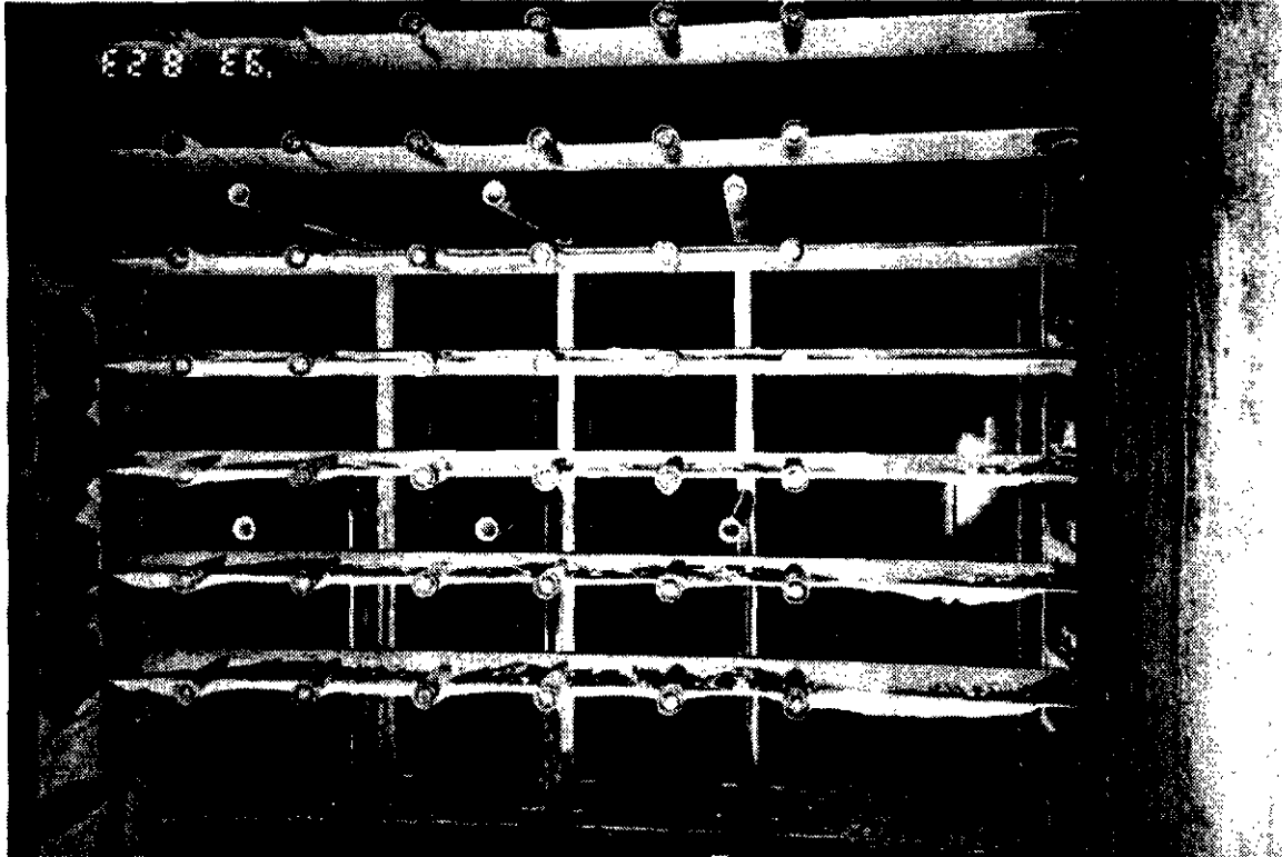
Figure 3-4. Humidification and Sorbent Injection Grids (East Half)
