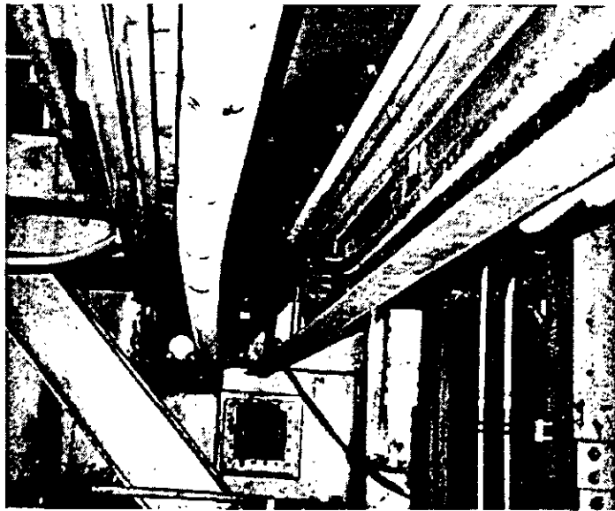
Figure 3-4. SNCR ARIL Bowed Lance
