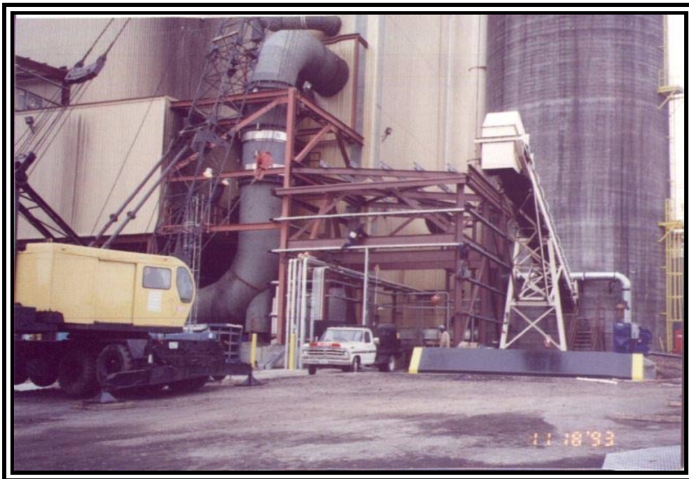
Figure 5.4: Drive-in Sump Under Construction.
