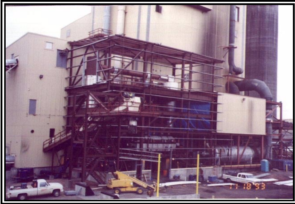
4.5b: PDF Deactivation System Under Construction.
