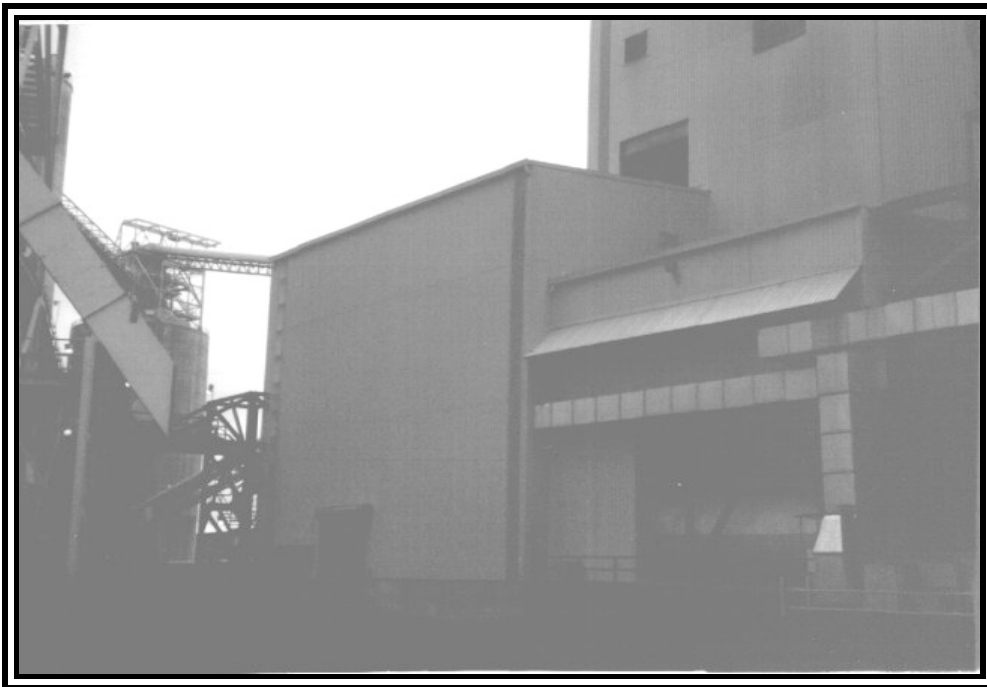
4.5c: PDF Deactivation Building Completed.
