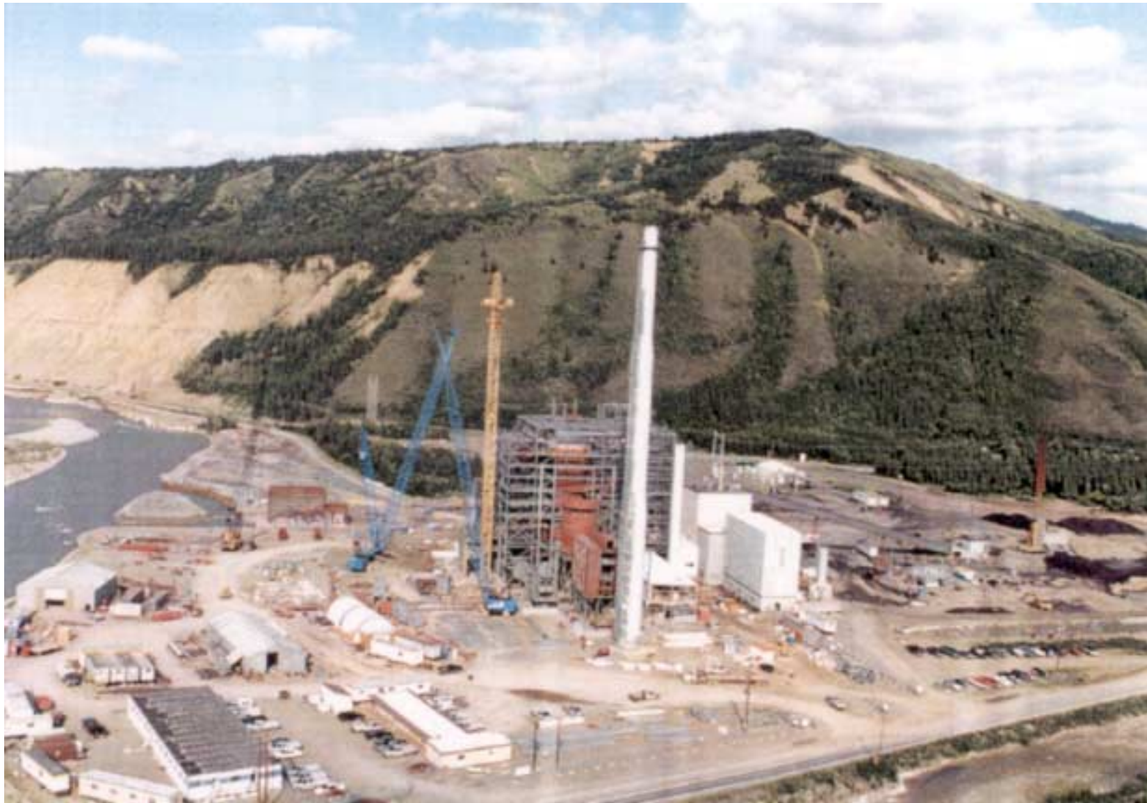
Figure 1-4 Site Construction Complete – 1997 (side view).
