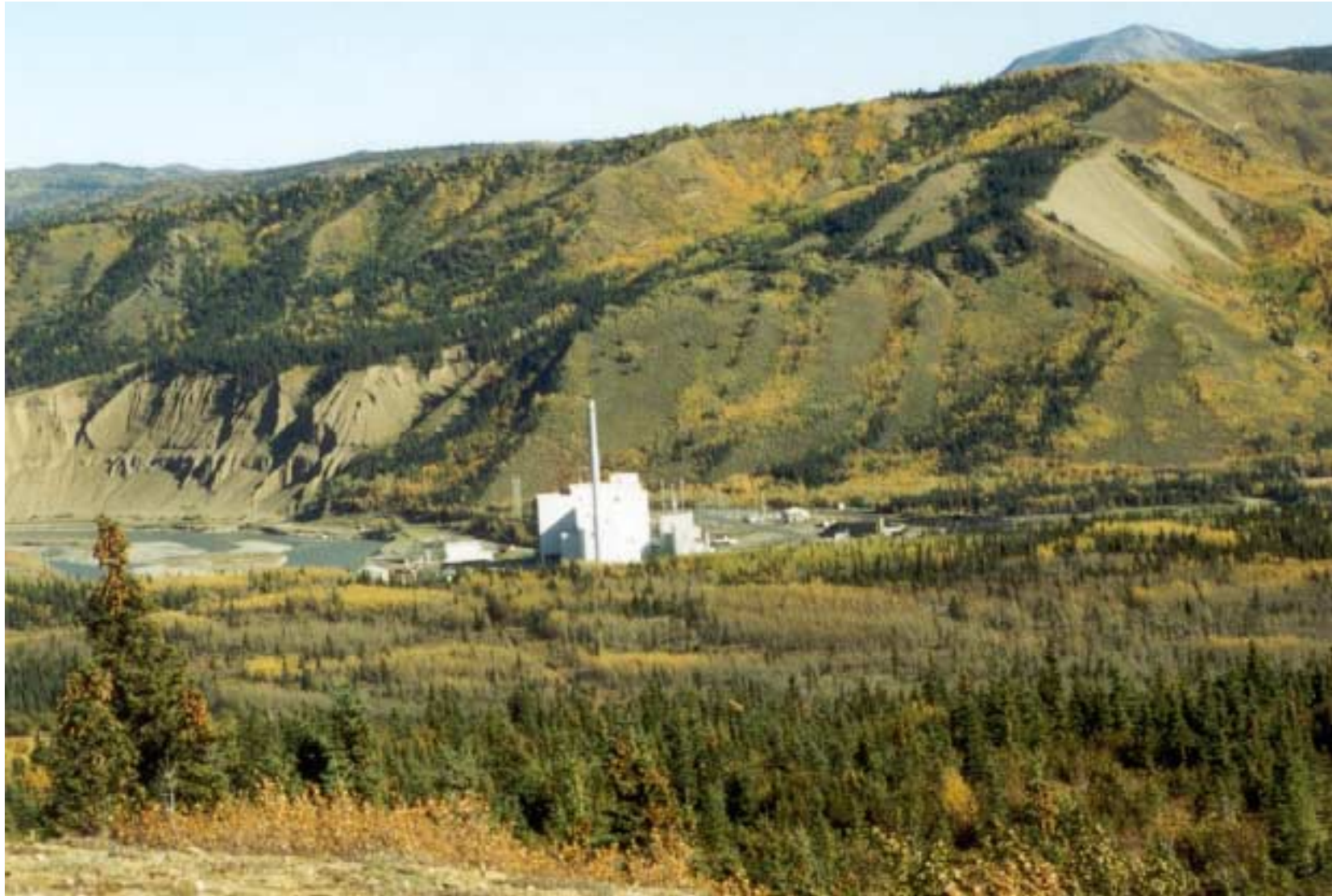
Figure 1-5 Site Construction Complete – 1998 (aerial view).
