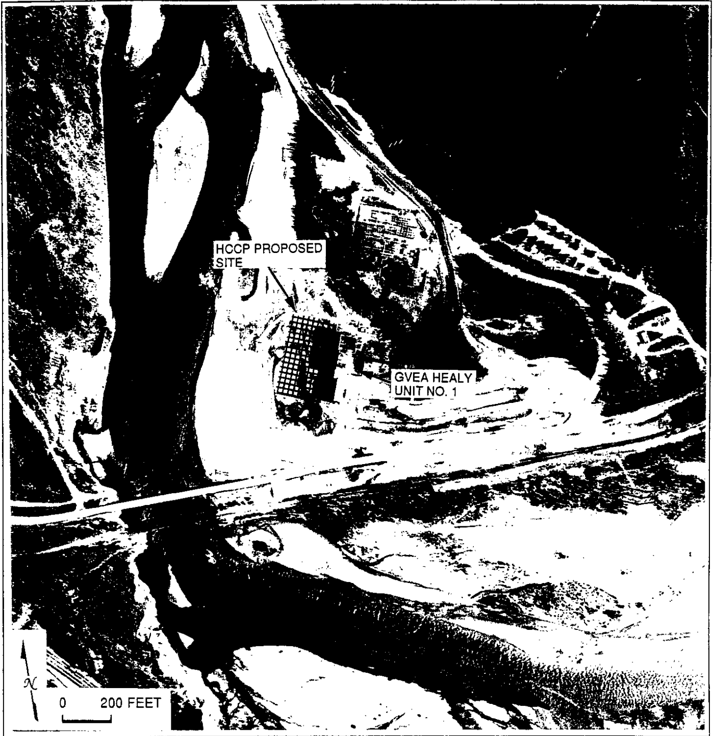
Fig. 3.1.3. Aerial view of the Healy Clean Coal Project proposed site.
