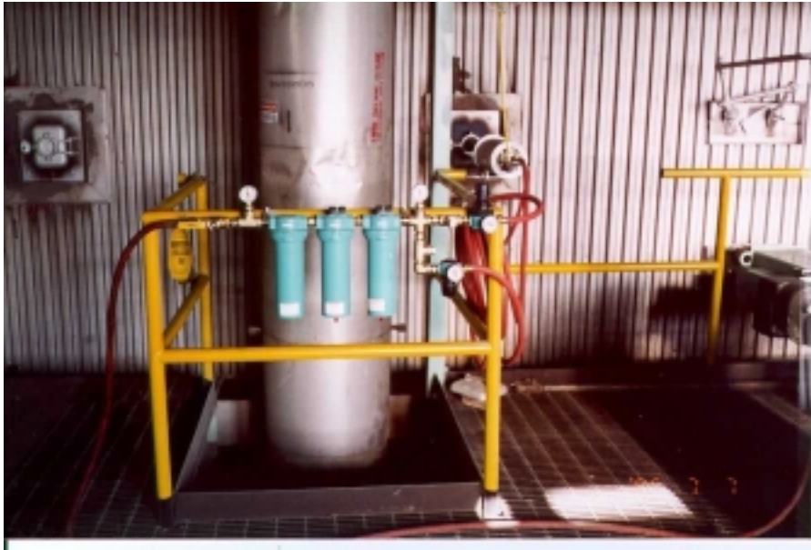
Figure 1 FOCUS Camera and Air Filter Assembly
