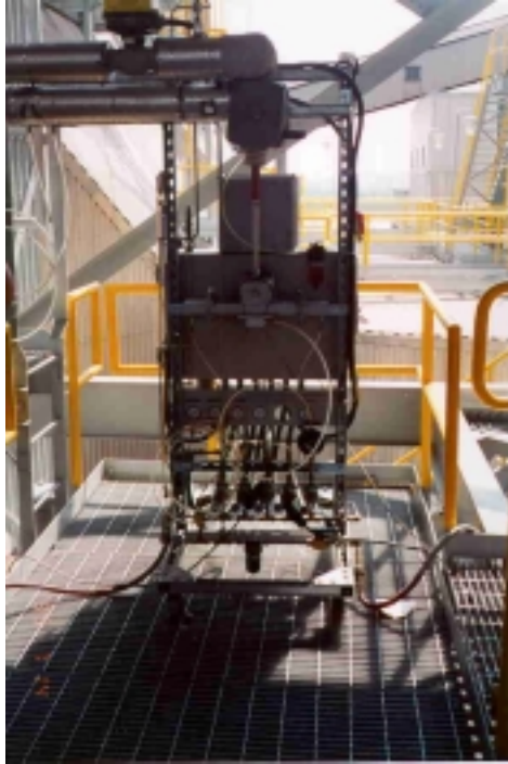
Figure 3 CAM Carbon-in-Ash Monitor (Rear View)
