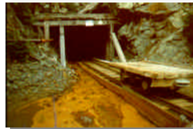
Contaminated Mine Drainage
