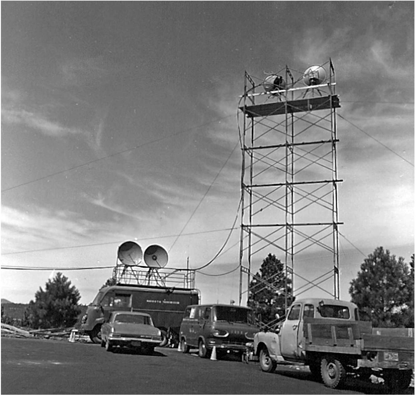
Figure 62-(m) television microwave relay towers set up behind the Center of Astrogeology headquarters building on McMillan Mesa for live TV broadcasts during Apollo 11; USGS photo P858PR, F76979.
