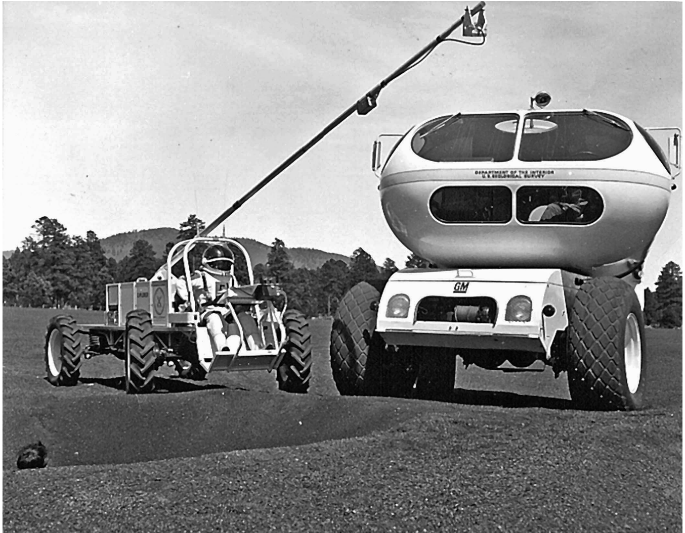
Figure 60-January 1969 field exercise at Cinder Lake Crater Field with MOLAB/MGL and Explorer vehicle for the National Geographic Society; (a) MOLAB and suited test subject on Explorer at Cinder Lake Crater Field for January 1969 exercise. Explorer vehicle had magnetometer boom attached; USGS photo P741, F16960PR
