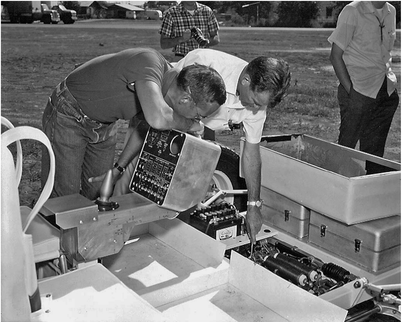
Figure 78-(c) Putty Mills (light shirt) showing power supply for electric motors that drive wheel to Charles Duke; USGS photo
