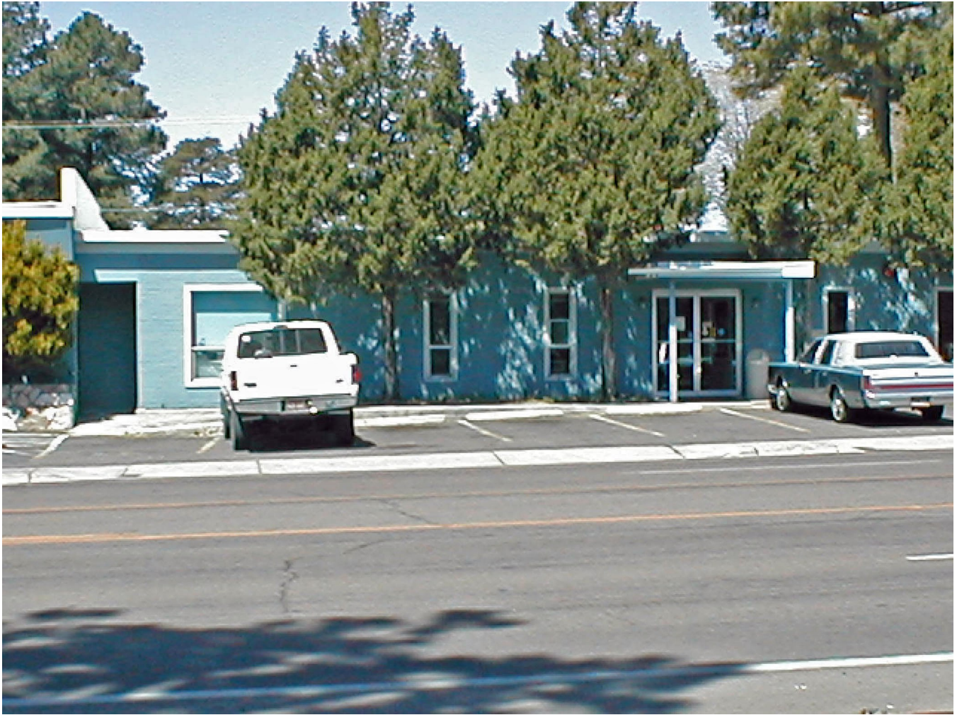
Figure 44-(b) second, larger, building (2717 N. Fourth Street) built adjacent to the ADF (2717 N. Fourth Street) at the same time to house some of the Branch support groups, including photogrammetry, surveying, photography, and cartography from late 1967 through 1973; digital photo by G. Schaber 6 may 2002.
