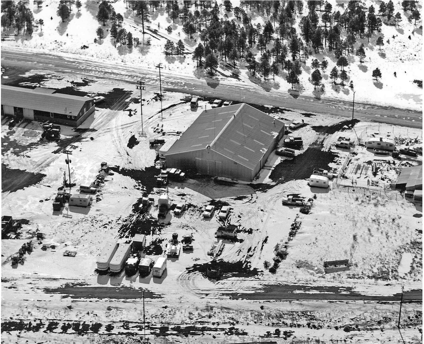
Figure 45-Construction phases of the Branch of Astrogeology's lunar Roving vehicle (LRV) called "Explorer;" (a) aerial view of the old Byrd Building at 1980 Huntington Road in Flagstaff, Arizona where the Branch of Astrogeology's "Explorer" simulated Lunar Roving Vehicle (LRV) was designed and constructed in spring 1967 by Putty Mills, Dick Wisner and Bill Tinnin of the Branch's Field Test Support Group in Flagstaff; USGS aerial photo
