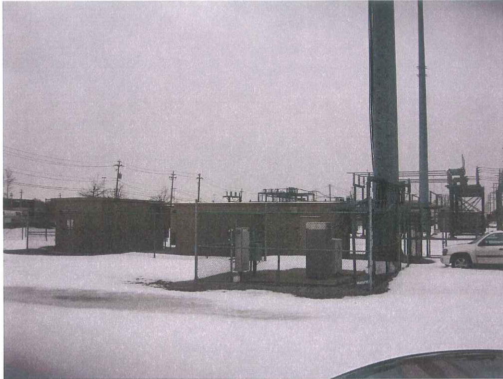
Plate 7: Verizon CLE457 - Dismissed ~190-foot monopole 41-28-35.8, 81-53-47.8 Sperry & Clague Roads, Westlake, Ohio
