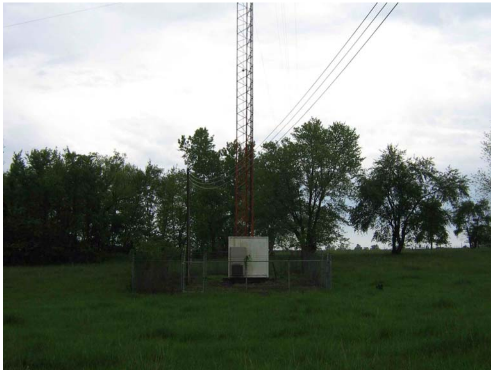
PHOTO 2: VIEW OF SITE, FACING SOUTH.
